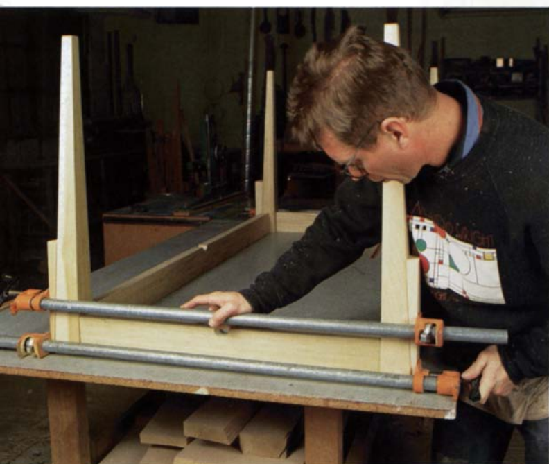
Two short rails connect the long-rail assemblies to complete the base. Adjust the clamping pressure above and below the tenon locations to keep the shoulders tight against the legs.
