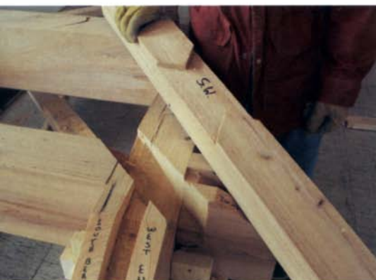
When carpentry is cabinetry. Some of the traditional Japanese joinery in the cypress bell tower by Grey Doffin and Jeff Kern looks as if it's been borrowed from furnituremaking.
