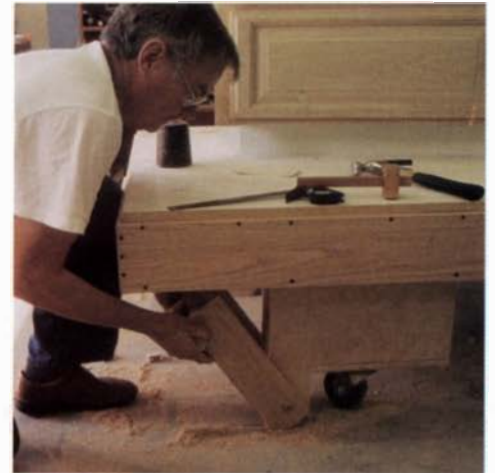
Building a low, mobile assembly table, p. 38
