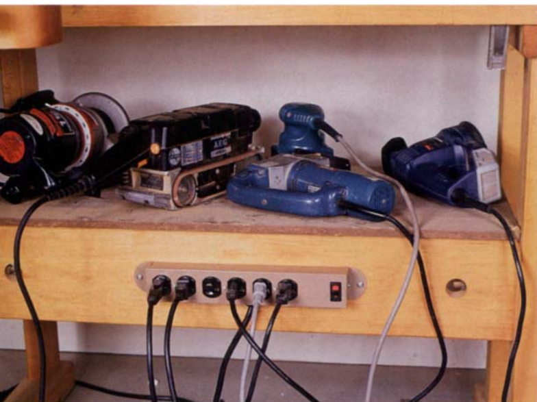
A multiple-outlet power strip is an economical way to add extra outlets to a workbench, and it speeds up work because you can leave several portable power tools plugged in at a time. Most power strips have a built-in circuit breaker, in case there's an overload.
