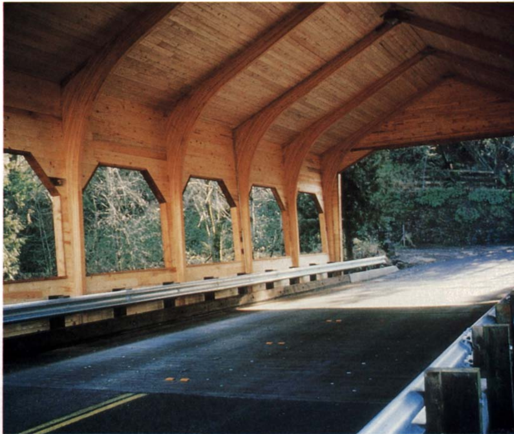
Multnomah County's (Ore.) covered bridge, of prefab arched gluelam fir with cedar.
