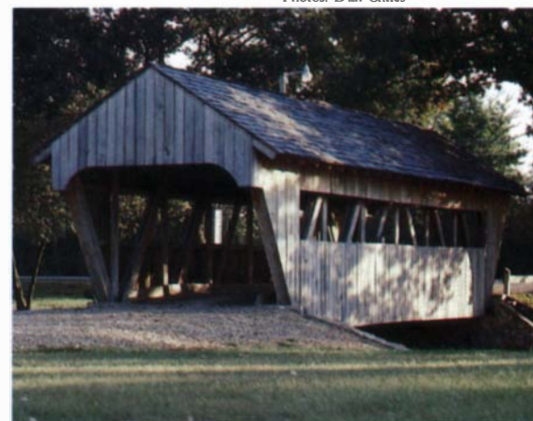
Chiles' multiple king-post bridge.
