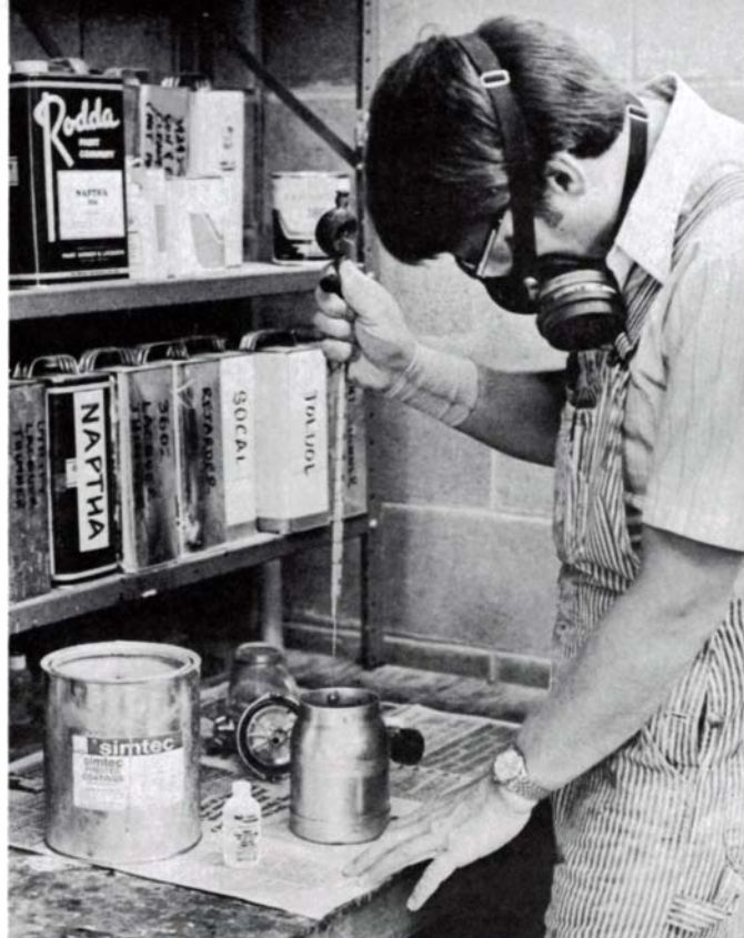
Polyester catalyst is toxic and extremely flammable. To avoid splashing it, Steinert adds it to the resin with a glass pipette, available from laboratory supply houses.
