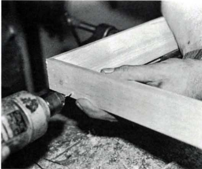
Predrilling nail holes guards against splitting, ensures good starts in the right direction for maximum purchase. One side of the frame is held in a machinists' vise, the other is steadied from underneath by hand, the forearm resting on something solid.
