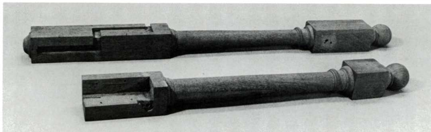
The landing newel (top) and starting newel, with their housings. Note the difference in the lengths of the turned shaft and of the square sections.
