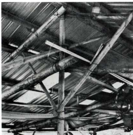
Brackett's pole-and-wire shop is spacious and well ventilated; detail, left, shows cross-bracing at central post.
