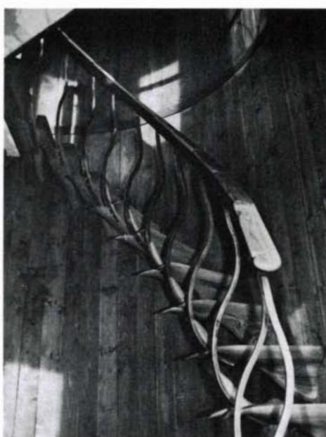
Willner buried two threaded rods inside the deep keel of each carved tread on this staircase. The rods are bolted through steel plates on the outside of the silo wall.
