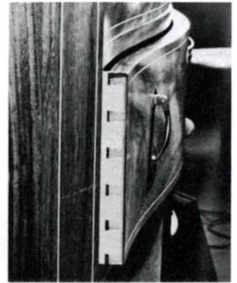
Drawer detail from tall chest (shown on next page). The serpentine front is laminated from four layers of \frac{1}{8} -in. oak, with thick rosewood veneers front and back, for dimensional stability. The back veneer is apparent at the wide end of the dovetail pins. A slice of rosewood was glued to the top edge of the oak core stock before the plank was resawn into laminates for bending—a nice solution to a difficult problem.
