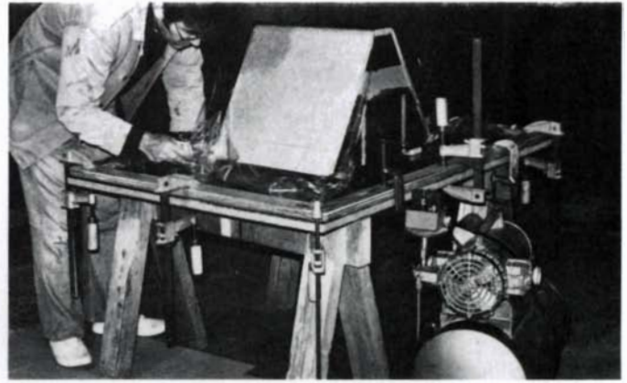
2 Bag is smoothed over workpiece in dry run. Tucking excess blanket neatly around form prevents blockage of air outlet.
