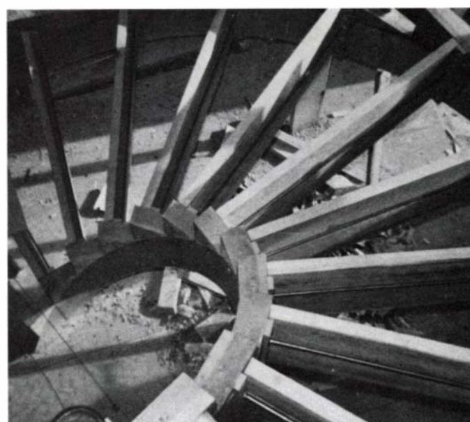
Done with laminating, Gigacz adds horizontal tie-members reinforced by iron rod, and step-forming blocks, and removes the forming cylinders. The stairway is on its own.
