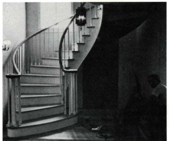
Author finishes trim on circular staircase, which is supported only at the floor and landing. The sweeping railing was laminated on the same forms as the stringers, then carved to shape by hand.
