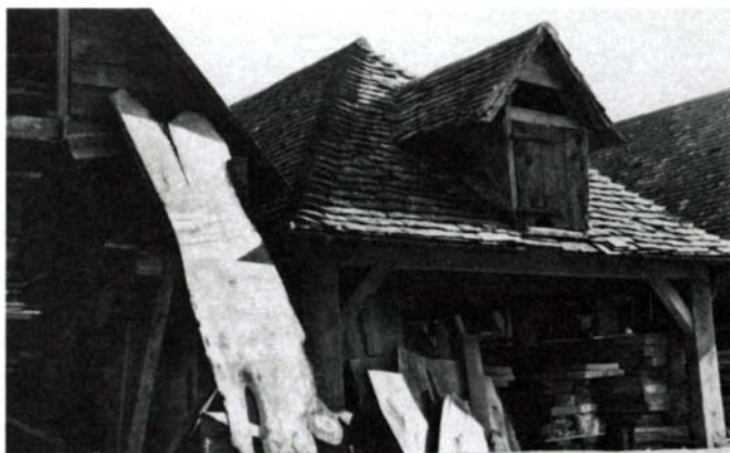
This lumber shed was built by Geoffrey Lupton around 1900 on what is now the Barnsley property; Barnsley has since added four more sheds of similar size. The locally cut wood is stickered to air-dry for five years per inch of thickness.
