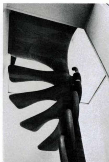
Treads of this closet stairway fit over a steel pipe bolted to the concrete basement floor. Individual handholds eliminate railing. Material is red oak.
