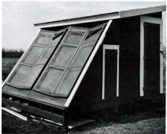
Solar panels on Johnson's kiln are tilted to catch early morning and late afternoon rays. Small door gives access to rear of solar collector, large door to stickered lumber.
