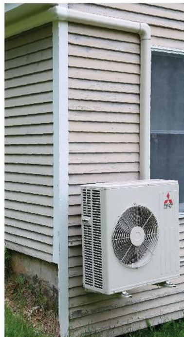
Strategically placed. Because of the outdoor compressor, the air handler is best placed on an exterior wall to simplify installation. Also, since the outdoor unit is exposed to the elements, it needs to be off the ground. If it snows in your area, the unit must be above the anticipated snow level and under a roof that still allows for ventilation. If it gets buried, it could stop functioning.
