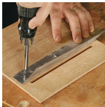
Let air sweep the floor. A thin plywood panel blocks all of the louver slots in the access door, except the lowest. That slot is still several inches above the new floor, so install a sheet-metal louver to direct incoming air down to the floor. Attach the panel with construction adhesive.
