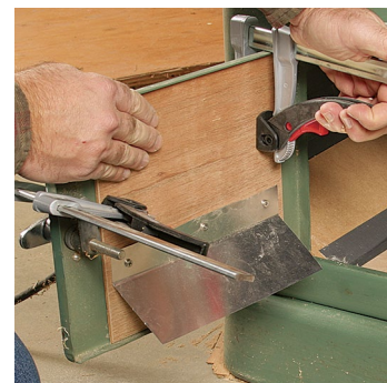
Let air sweep the floor. A thin plywood panel blocks all of the louver slots in the access door, except the lowest. That slot is still several inches above the new floor, so install a sheet-metal louver to direct incoming air down to the floor. Attach the panel with construction adhesive.
