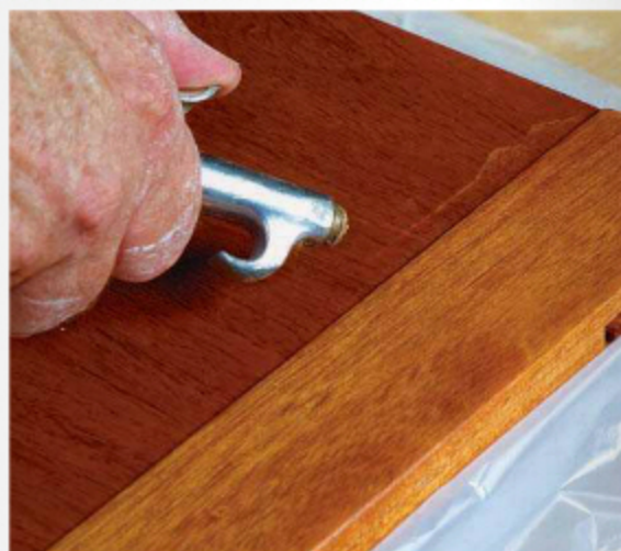
No place for surplus varnish to hide. No matter how much you wipe, varnish has a habit of oozing out of joints after you have done your final buffing, creating sticky and glossy areas. Remove surplus varnish using compressed air, and wipe the area clean.
