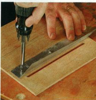
Let air sweep the floor. A thin plywood panel blocks all of the louver slots in the access door, except the lowest. Because that slot is still several inches above the new floor, install a sheet-metal louver to direct incoming air down to the floor. Attach the panel with construction adhesive.
