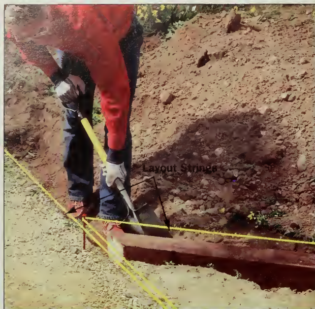
Figure 2: Excavate a level trench, making sure the first timber will be buried at least halfway for stability. String lines mark the rough outline of the retaining wall.
