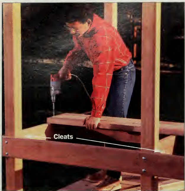
Figure 5: Attach decking with 3-inch weatherproof screws in pilot holes. Cleats are screwed on where extra support is needed.
