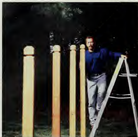
Figure 5: Check the posts to be sure they're plumb and square, and that the tops form an even line. Because the posts are set in dirt, you can adjust them if necessary.
