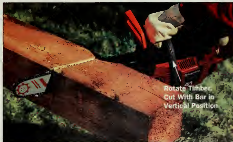
Figure C: Cut the timber with a chain saw. Turn the timber so that the chain saw bar is vertical when cutting. Coat the cut end with a liquid wood preservative.
