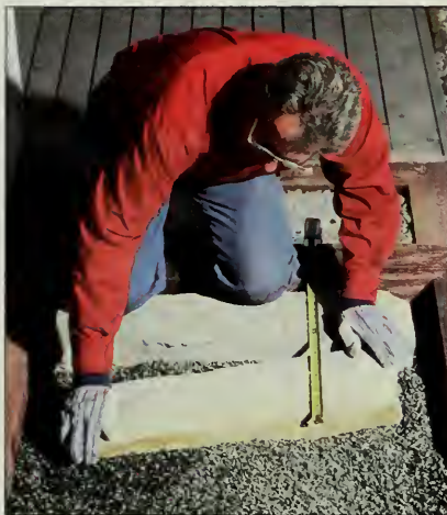
Figure 11: Set the tread into the fill rock by moving it in a back-and-forth, twisting motion. Recheck the tread height. If it's too high, twist it farther into the fill rock. If the tread's too low, add more fill rock under it.
