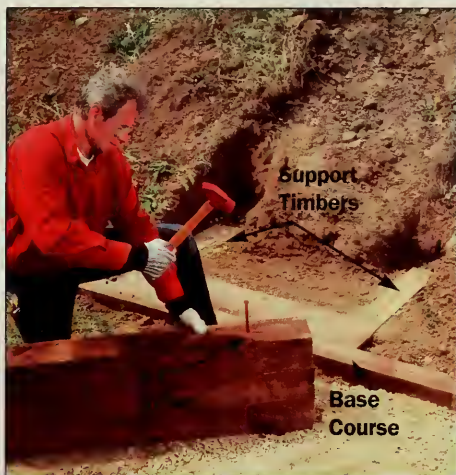
Figure 9: Spike together three timbers, keeping the top surface flat. Level support timbers (in background) for the next step unit to rest on.
