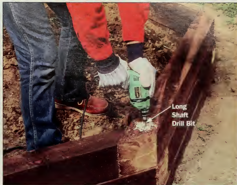
Figure 5: Predrill spike holes at corners to prevent splitting. Use a 12-inch long spade bit that's slightly thinner than the spike itself.
