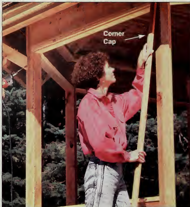
Figure 20: Install corner caps where the walls join.
