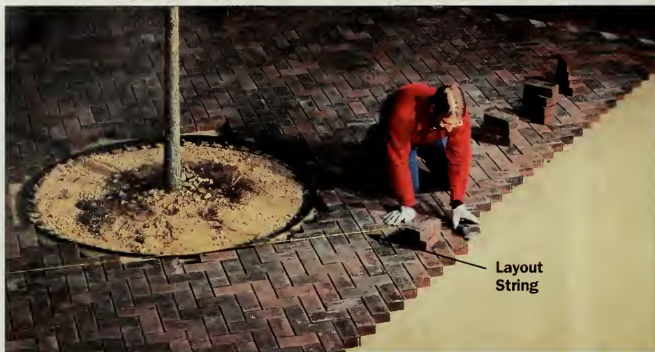
Figure 10: Continue laying pavers using a layout string to keep them in line as you work. Put a gap between pavers or tap them tighter to stay in line.
