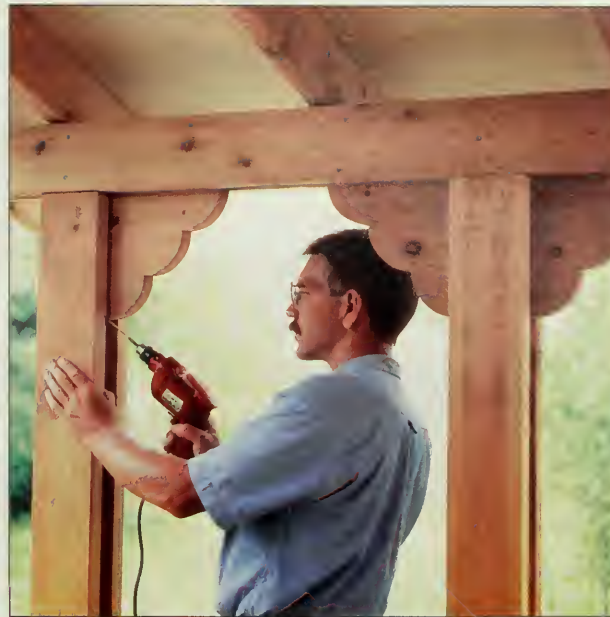
Figure 22: Fasten brackets in place to stabilize posts and beams. Paint, stain, or seal all exterior surfaces, and your shed is done.
