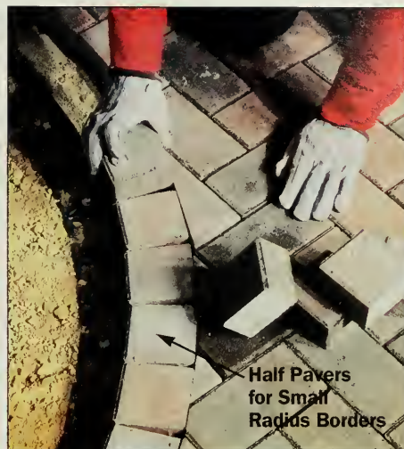
Figure 12: Use half pavers for bordering tight circles. Smaller pavers cut down on the size of the pie-shaped gaps between each piece.
