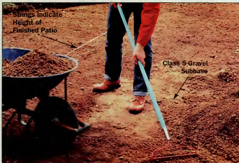
Figure 4: Spread class 5 subbase to a depth of 4 inches over the entire patio area and 8 inches beyond. Measure from the guide strings to obtain a uniform height.
