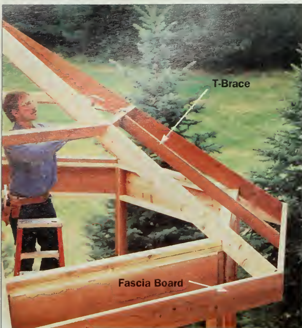
Figure 14: Install roof bracing, which is in the shape of a “T”, after nailing 2x8 fascia boards to the ends of the rafters.
