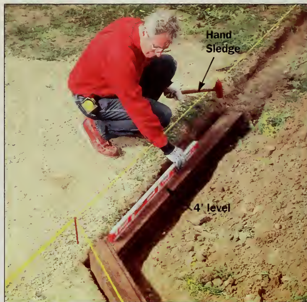
Figure 3: Install the first course of timbers, making certain they're level and resting on firmly packed earth. Use a hand sledge to help fine-tune timber height.
