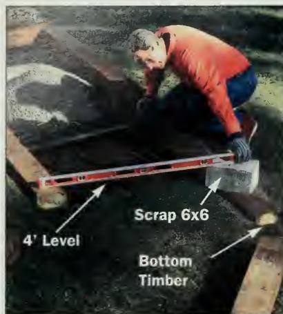
Figure 14: Check the level of the path's edge timbers. To make leveling easier, check each row of a double row of timbers. Use a piece of 6x6 under the 4-foot level.
