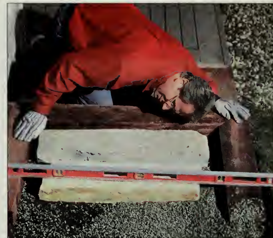
Figure 10: Place the step tread stones (wallstones) onto the layer of fill rock. Check the height of the tread surface against the height of the side timbers. The tread should be level with the timbers.
