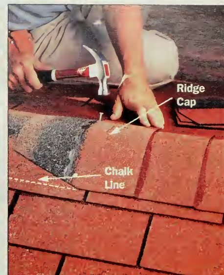
Figure 17: Install ridge cap. Individual shingle tabs with cut-off corners overlap one another to waterproof the ridge and give a finished appearance.
