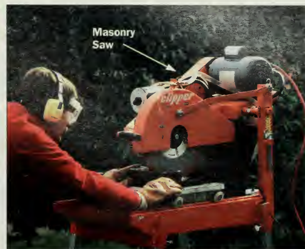
Figure 13: Cut pavers with a masonry saw. The saw has a built-in sliding carriage for moving pavers past the blade. Recirculating water keeps the blade cool and lubricated.
