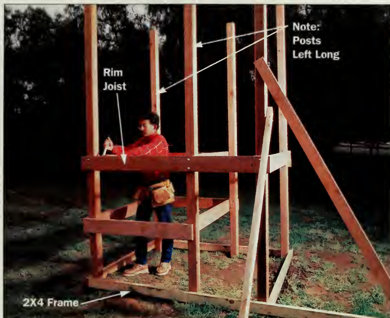
Figure 3: The remaining posts are held in position by a temporary frame of 2x4s. As posts are plumbed, attach the rim joists.
