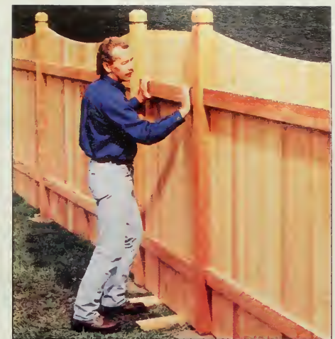
Figure 15: Twist the gate so the stringers line up with those on either side. Then finish nailing the boards and add a diagonal 2x4 brace pointing toward the bottom hinge.
