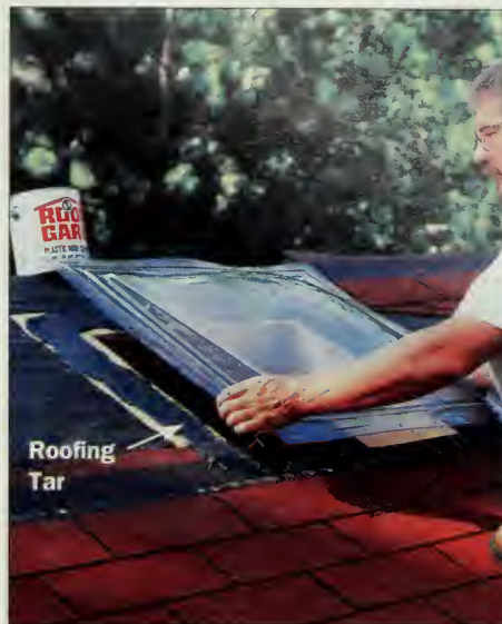
Figure 16: Install skylights, embedding them in roofing tar. Skylights located near the peak of the roof let in the most light.
