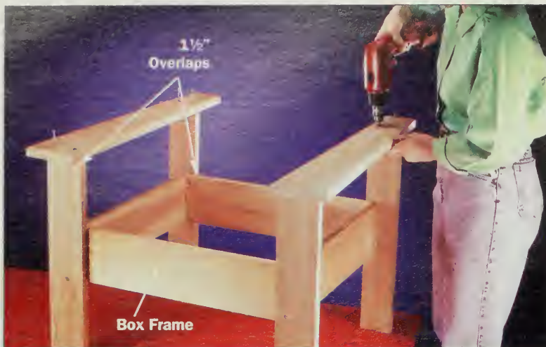
Figure 3: Screw the arms to the tops of the legs after attaching the legs to the box frame. Also use waterproof glue on all joints.
