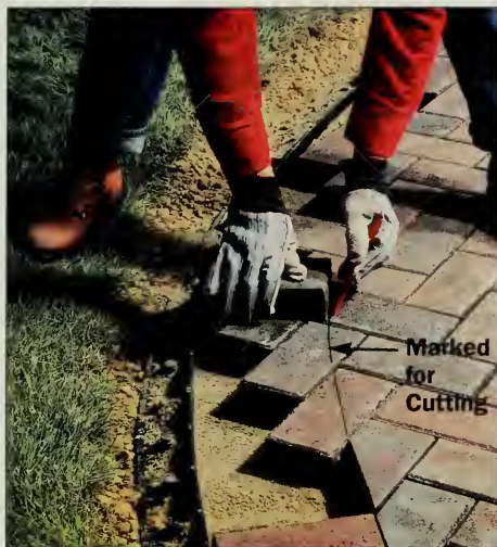
Figure 11: Mark pavers that run “wild” into the border area. Then remove the pavers, cut them to size, and place them back in position along with the border pavers.
