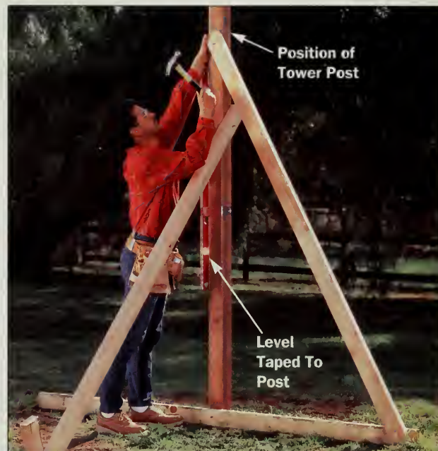
Figure 2: Brace the first post so it's plumb. Use screws or duplex nails for easy disassembly, and don't cut the posts to length yet.
