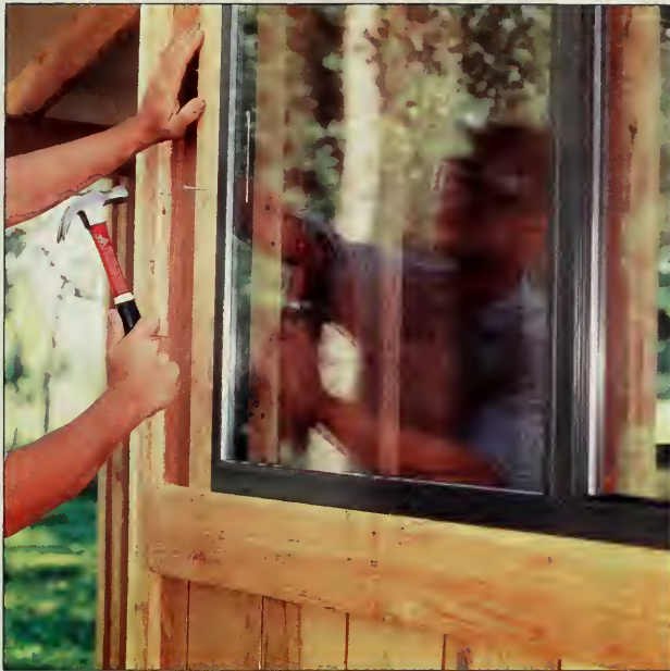
Figure 21: Install the windows and the cedar window trim. Horizontal 1x6 boards cover the siding seam and Z-flashing.
