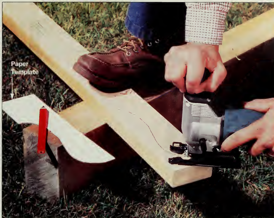
Figure 3: Cut rafter ends with a jigsaw, using a paper template to get the shape.
