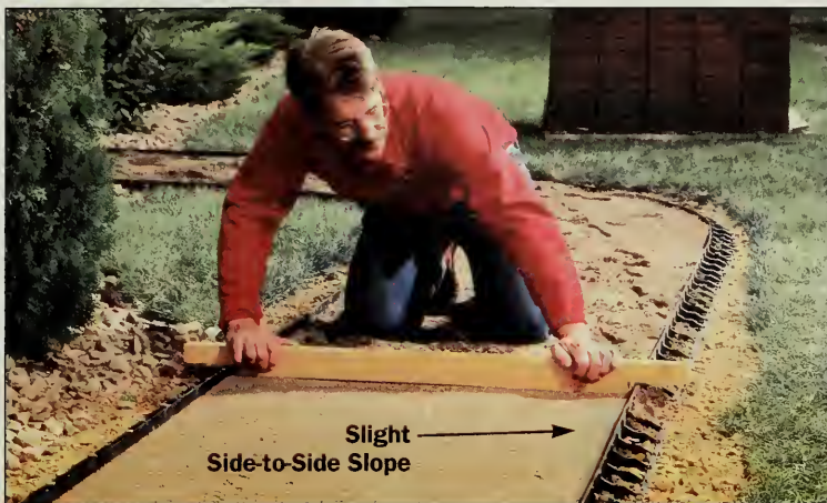
Figure A: Smooth and level the sand using a notched screed board riding along the edging for a guide. Include a slight tilt for good drainage.
