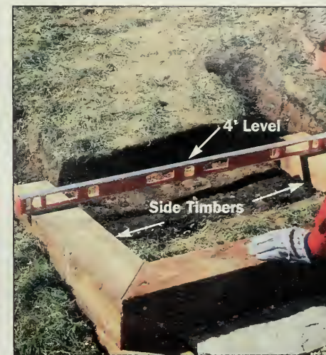
Figure 6: Check the side timbers for level by placing a 4-foot level across the step. Raise low timbers by adding fill rock under them.
