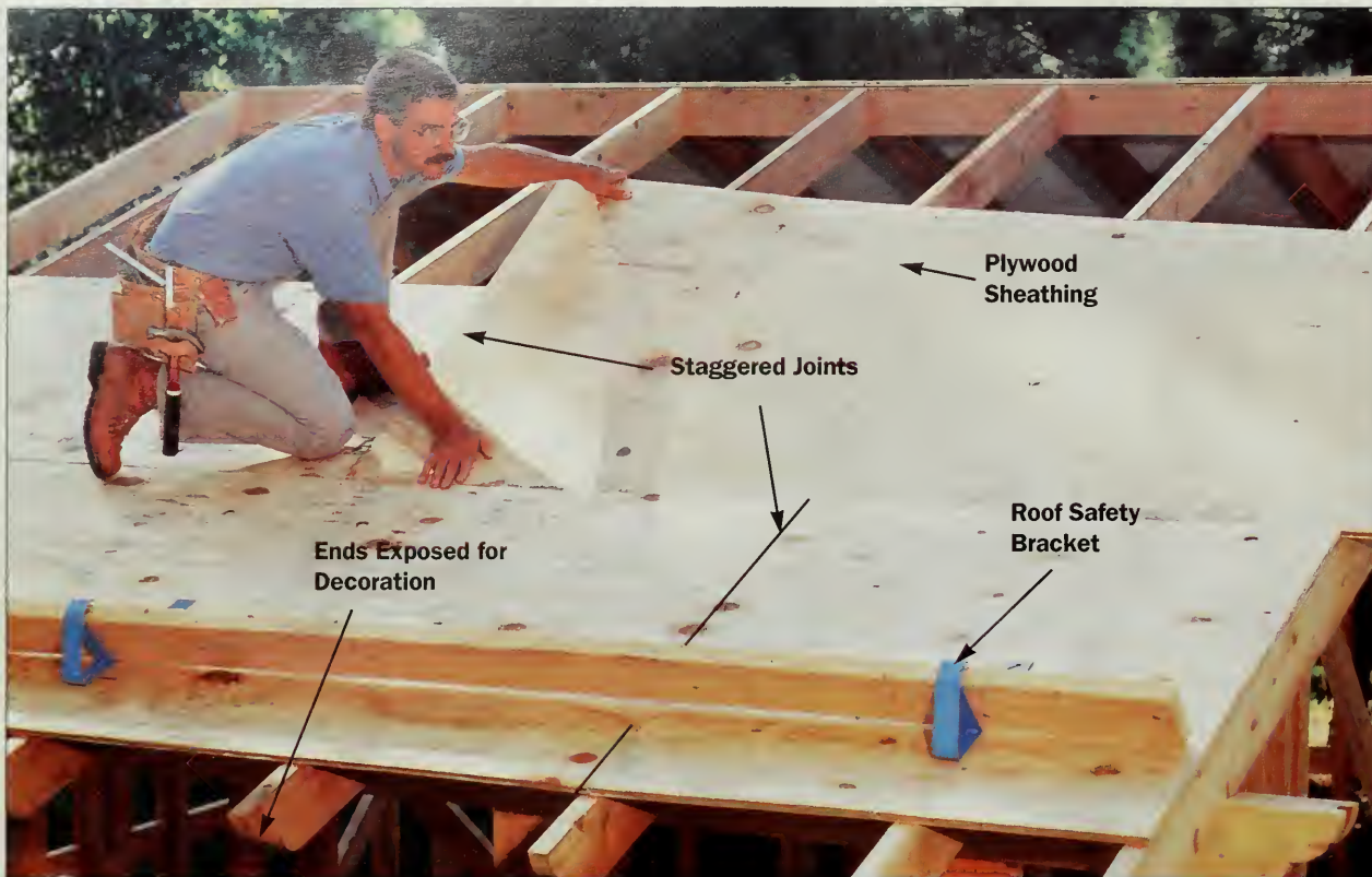
Figure 13: Install plywood roof sheathing, trimming excess plywood after nailing. Stagger end joints and nail securely with 8d nails.
