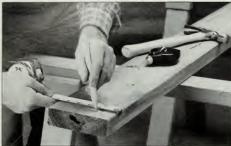
Figure 1: Mark the proper width at both ends of the deck board, AND in the middle if the board is warped. A chalk line marks the cut.
