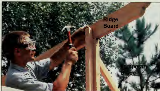
Figure 9: Install the ridge board on top of the support post. Decorative end cuts are quick and easy to make with a jigsaw.
