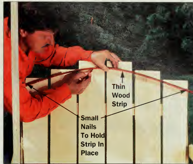
Figure 8: Mark the arc on the back slats using a thin strip of wood bent evenly between small nails near the edges of the outside slats. Unbolt the back and cut the arc with a jigsaw.
