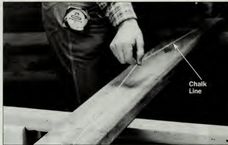
Figure 2: Hook the chalk line at one end, stretch it tightly, lift the center straight up and let it snap down to leave a perfectly straight line.
