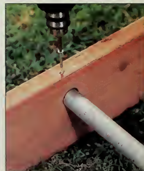
Figure 7: The monkey bars are pinned into the 2x6 rails by drilling a pilot hole and then driving in a 3-inch screw from the top side.
