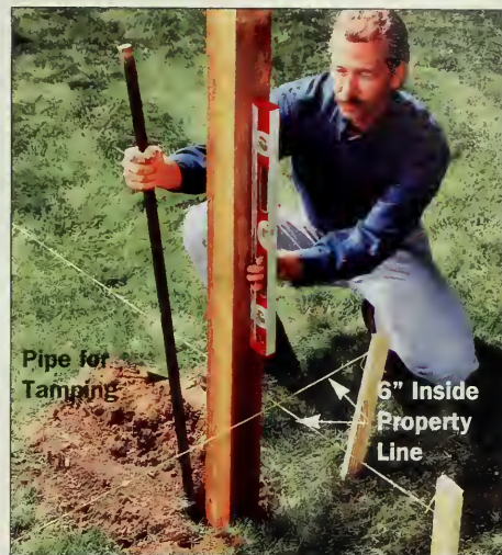
Figure 2: Tamp 6 to 8 inches of dirt around the corner posts, doing an inch or two at a time. Make sure the post is plumb and the right height.
