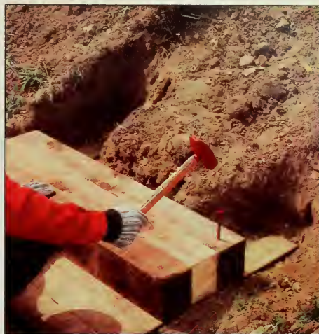
Figure 10: Secure triple-step unit in place by spiking it to the support timbers. Upper step overlaps the lower step approximately 2 to 3 inches.
