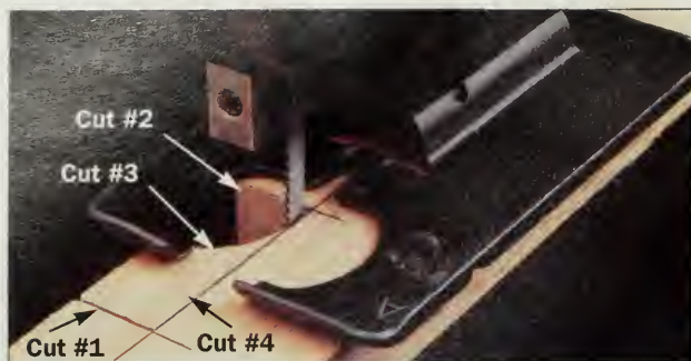
Figure 7: Cut 1x4 notches in the back supports using a jigsaw. The easiest way is to make four cuts in the order shown.
