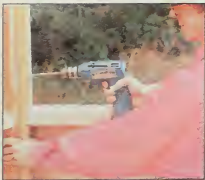
Figure 8: Fasten wall sections together with 3½-inch galvanized screws. If the studs don't meet perfectly, clamp them tight first.
