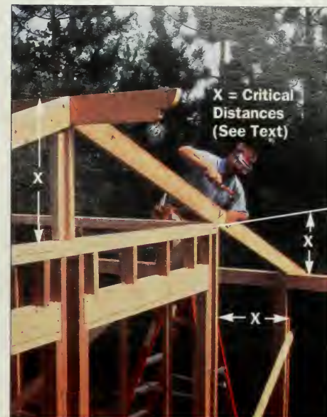
Figure 12: Nail rafters in place, installing the gable-end ones first. Space rafters every 2 feet and toenail them to beam and wall with 16d nails.
