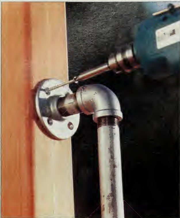
Figure 12: Handrails that kids can grip are assembled from 3/4-inch galvanized pipe and screwed to the wooden structure.
