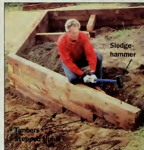
Figure 8: Step up hills by using progressively longer courses of timbers. Make sure timbers remain level as they reach from timber onto soil.
