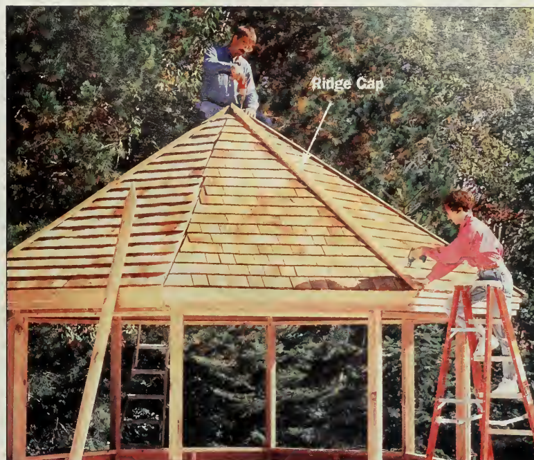
Figure 17: Screw ridge caps along the roof seams with galvanized deck screws. Ridge caps are cut at a 15-degree angle from 4x4 cedar posts (see plan detail, page 79).
