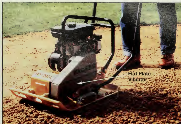
Figure 5: Tamp the subbase using a rented flat-plate vibrator. Work in a circular motion and compact the area twice.
