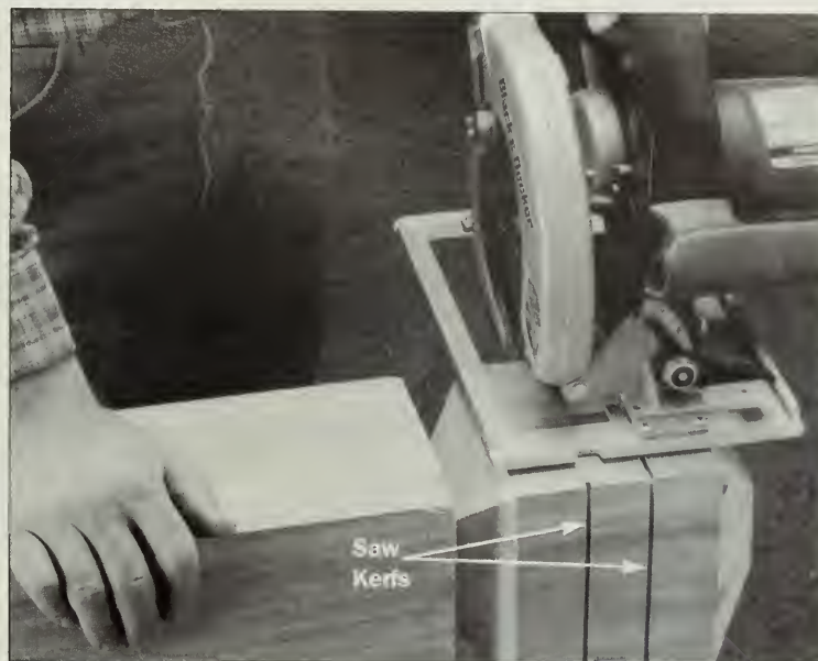
Figure 2: As you rotate the post, saw toward the previous cuts to avoid splintering the edges. Observe safe saw practices.
