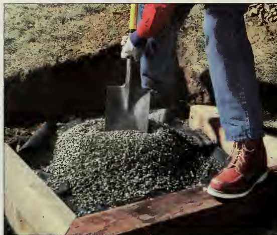
Figure 9: Spread an even, 1½- to 2-inch-thick layer of fill rock over the fabric. This is the same rock that's used to fill the gaps between the flagstone and timbers.
