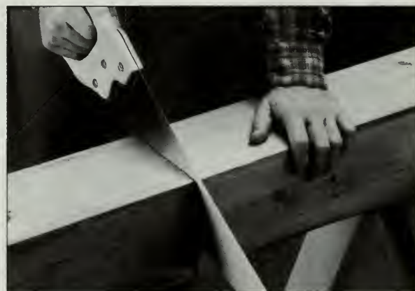
Figure 3: Complete the cut with a hand saw, since the power saw blade won't reach the center of a 6x6 post.
