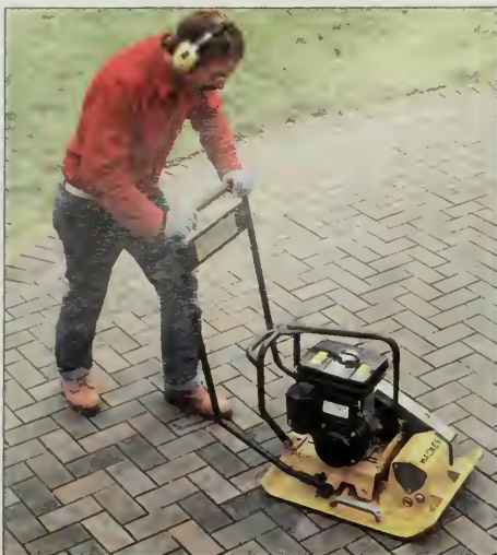
Figure 14: Tamp the patio with a flat-plate vibrator after all the pavers are installed. Tamp the entire outside edge first, then circle in.
