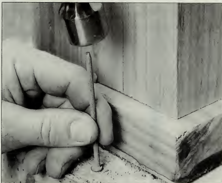
Figure 1: Blunt the nail by tapping its sharp point with a hammer, so the wood won't split when nailing close to the edge.
