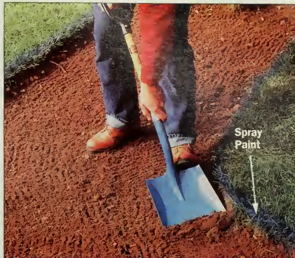
Figure 2: Remove sod in an area extending 8 inches beyond the boundaries of the patio. Spray paint indicates the excavation line.
