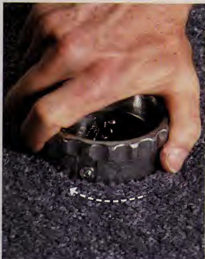
Cut out the stain. Twist to slice out the damaged area. Do the same in a closet to cut a perfect patch.
