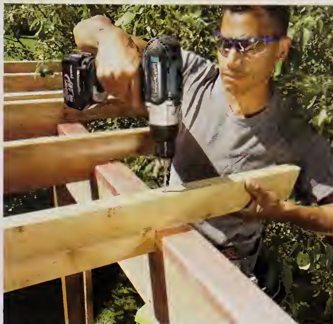
8 Set the rafters. The notches automatically set the rafters' overhang. Predrill and fasten each rafter end with a single 5-in. screw.
