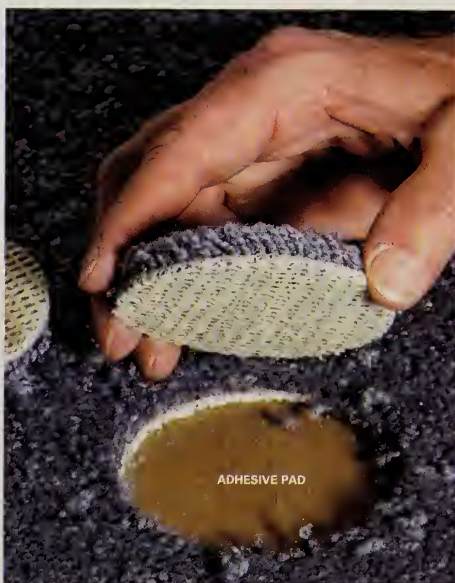
Stick in the patch. Lay in an adhesive-backed pad to secure the carpet patch. Make sure the nap direction of the patch matches the nap of the surrounding carpet.
