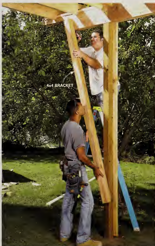
9 Add the brackets. Hold the 4x4 bracket in place and have a helper mark it along the beam and the post. Cut the bracket, screw it into place and add the second side of cladding.
