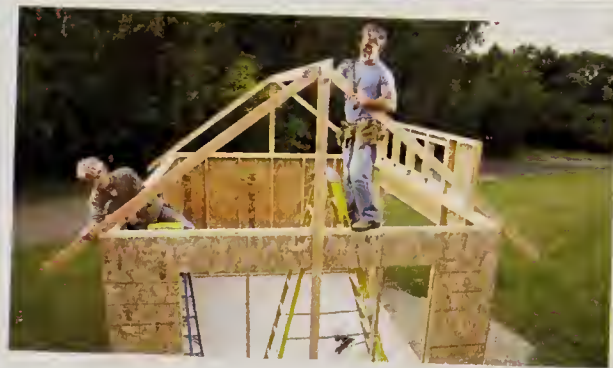
Framing the roof
