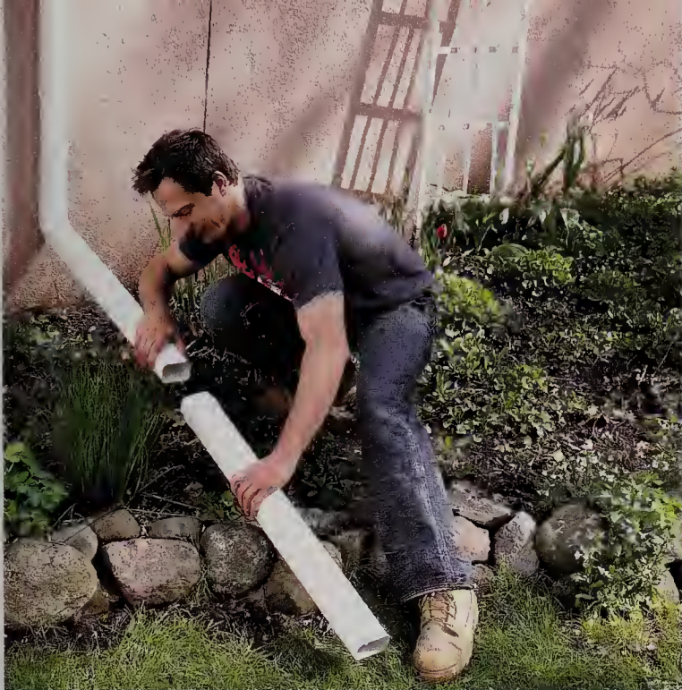
Downspouts should discharge water at least 10 ft. from the house. If yours don't, consider adding extensions.
