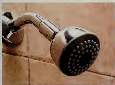
Replace showerheads and tub spouts with anti-scald fixtures to avoid dangerously hot water.
