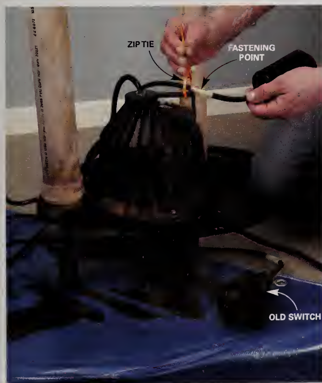
2 Use a plastic zip tie to attach the new switch cord to the pump at the same point the old cord was attached.
