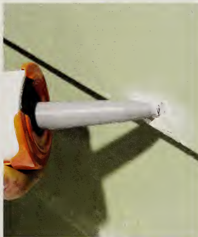
3 FILL the hole with acrylic latex caulk and smooth it with your finger. After the caulk skins over, repaint.
