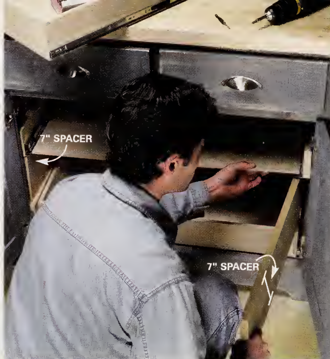
12 CUT plywood spacers to temporarily support the upper rollout and set them onto the carrier below. Rest the second carrier on the spacers and install it as shown in Photo 11.
