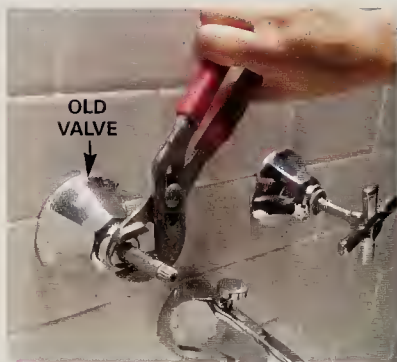
Unscrew the old handles. Mark the cover hole on the tile and cut it out with an abrasive blade in a jigsaw.
