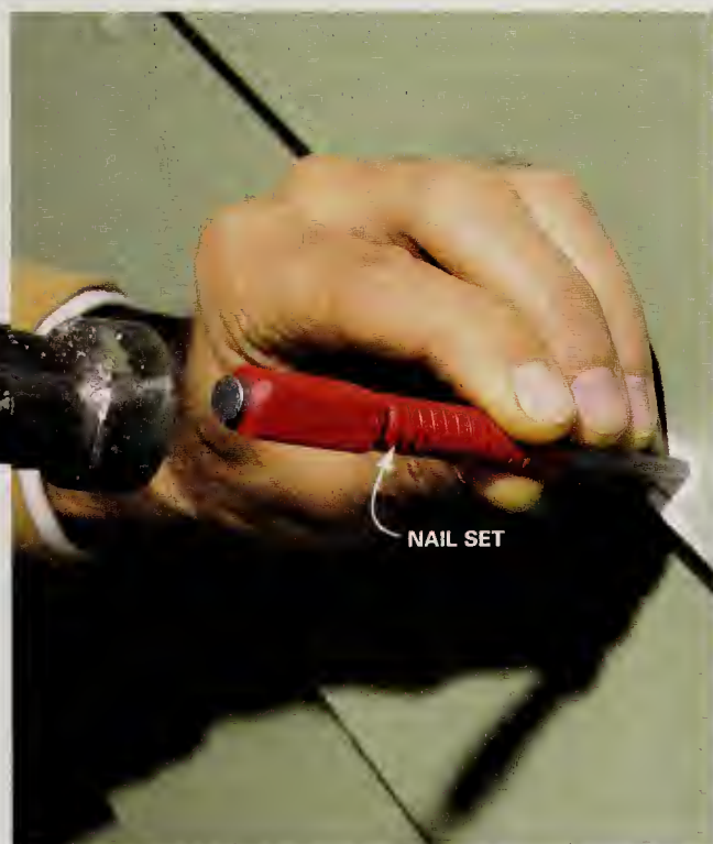
2 SET the nail about 1/16 in. below the surface and prime with a quick-drying, stain-blocking primer.
