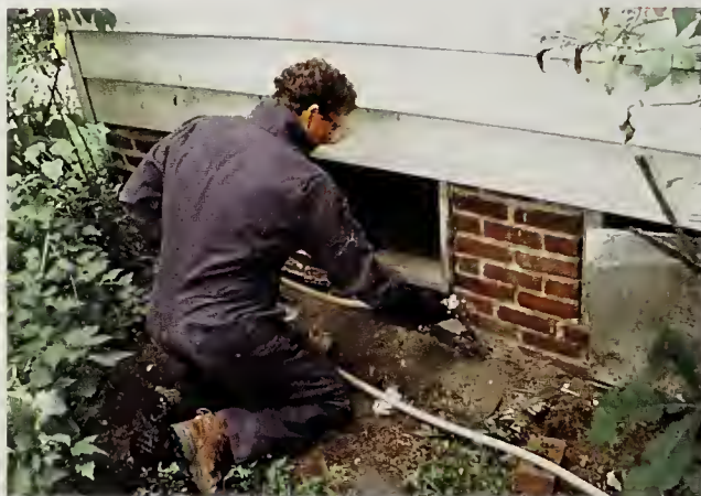
EXTERMINATORS don't just spray pesticides on surfaces. For effective, lasting treatment, they often drill holes and inject chemicals into wood, soil or masonry.
