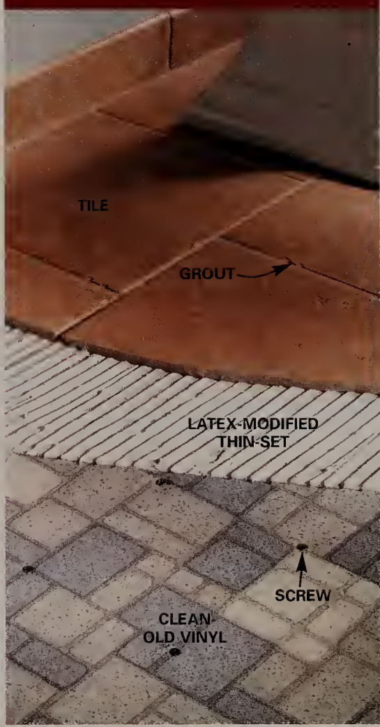
Method 2: Tile without underlayment
