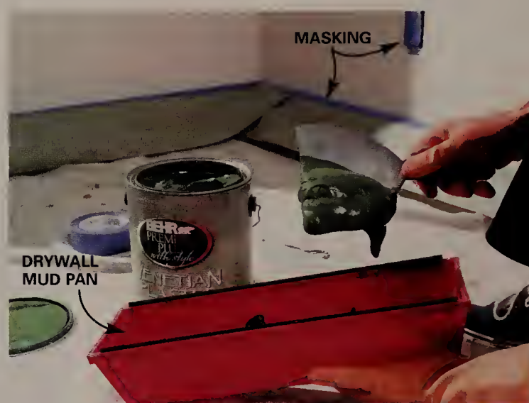
2 TRANSFER the Venetian plaster mix to a drywall pan so it's easier to scrape the excess off the knife. The plaster is a bit thinner than drywall compound but thicker than paint.
