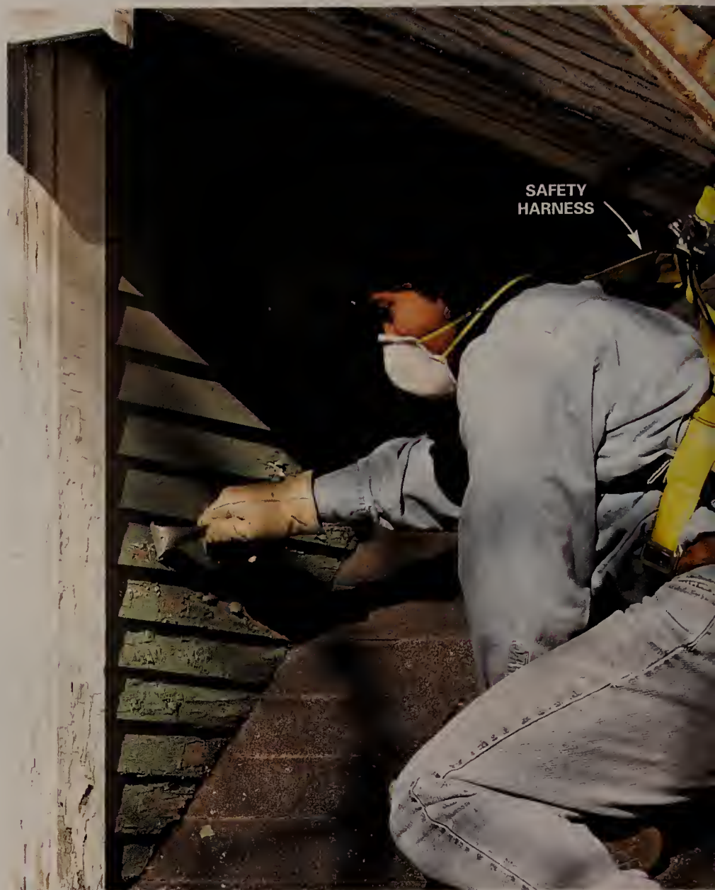
1 SCRAPE and sand to remove all paint from the area that's peeled. Keep a nail set handy so you can reset any protruding nails.
