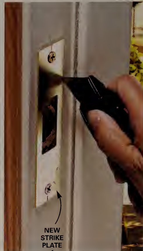
2 ALIGN new strike faceplate on the jamb, predrill screw holes and attach it. Score around the inner and outer edges with a utility knife. Remove the faceplate.
