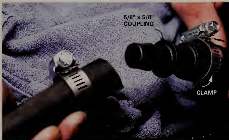
Push the hose firmly onto the coupling
