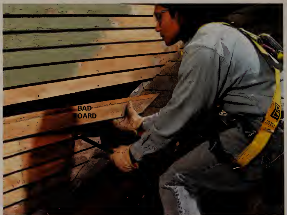
2 TEAR off any cracked or rotted siding, using a cat's paw and pry bar. Cut nails above bad boards using the technique shown in Photo 2, p. 193.
