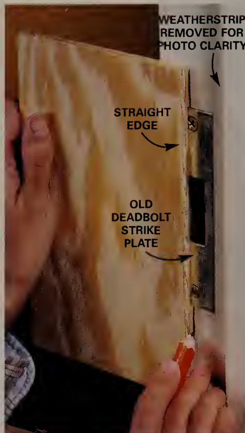
1 MARK the center of the existing deadbolt hole. Then remove the old strike plate.
