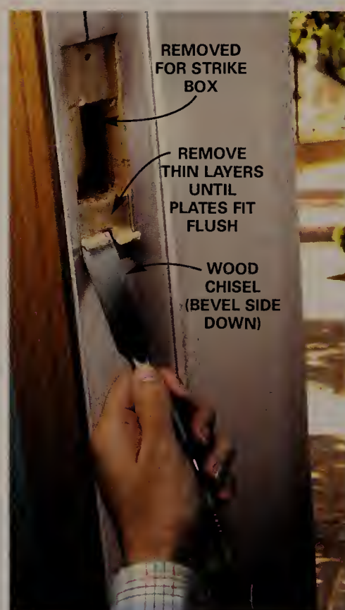
4 CHISEL OUT the strike box and strike plate areas so the strike plate will fit flush with the doorjamb surface.
