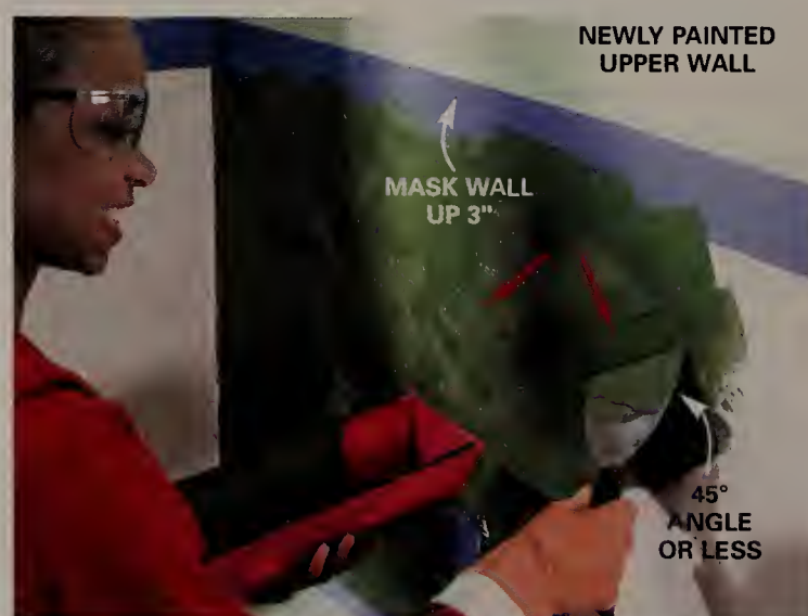
3 APPLY the colored plaster mix with your drywall knife in random strokes back and forth at less than 45 degrees to vertical. Avoid heavy buildup.
