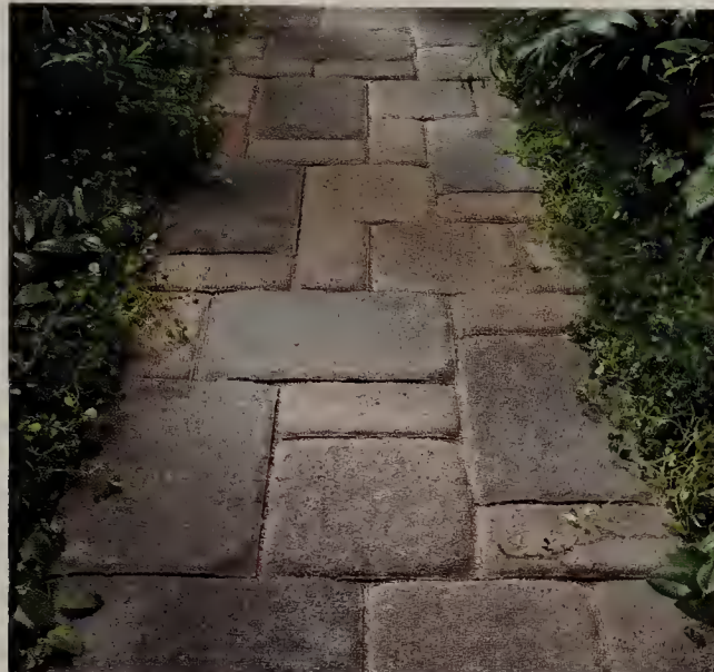
2 CONCRETE pavers are cast in a wide variety of geometric shapes and colors. Most have rounded edges.
