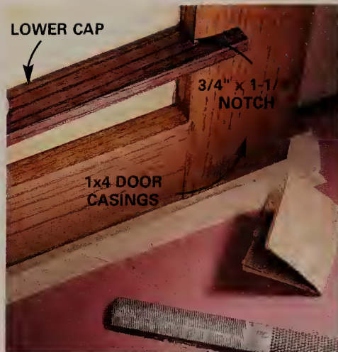
8 NOTCH the lower cap to overlap the casing by 1-1/4 in. Cut the notches a little undersized with a handsaw and file and sand to the lines.
