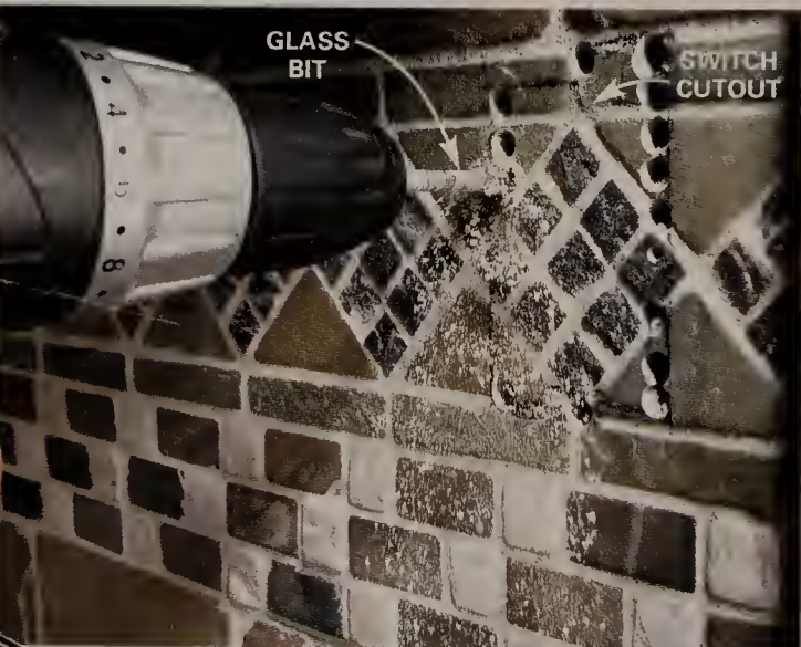
11 MARK the switch box profile on the backsplash. Drill a series of holes with a glass bit and chip out the tile and wallboard.
