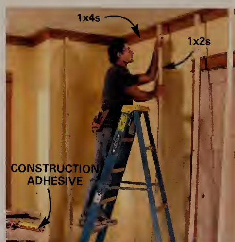
12 ALONG walls without ceiling framing, use construction adhesive and temporary braces to attach the boards.
