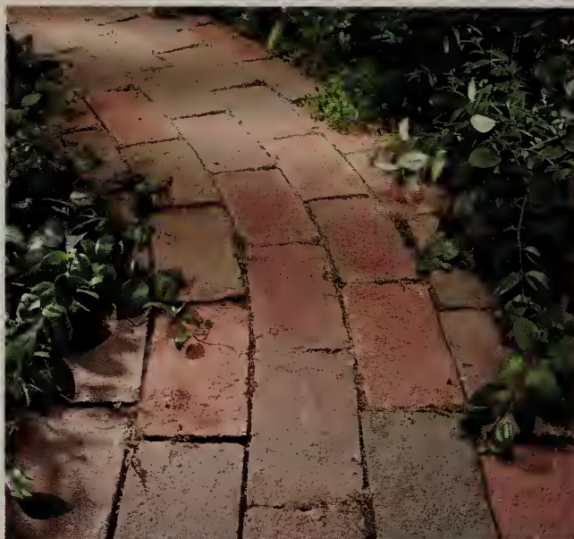
3 CLAY pavers offer the traditional brick look. Most have crisp, square edges.
