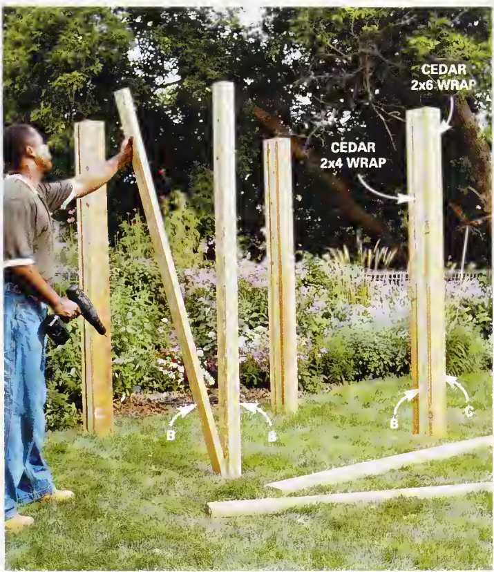
5 Wrap all sides of the pressure-treated 2x4s with cedar. Screw 2x4 cedar on the open sides of the posts and 2x6 on the bench sides of the posts using 3-in. deck screws. Be sure the tops of all the pieces are flush.
