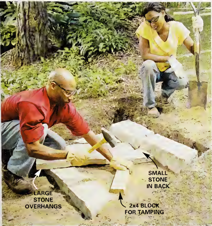
6 Arrange large flagstones to overhang the lower riser about 2 in. Remove soil or tamp gravel into low areas to level the tops of the stones. You can leave gaps between stones up to 2 in. wide.
