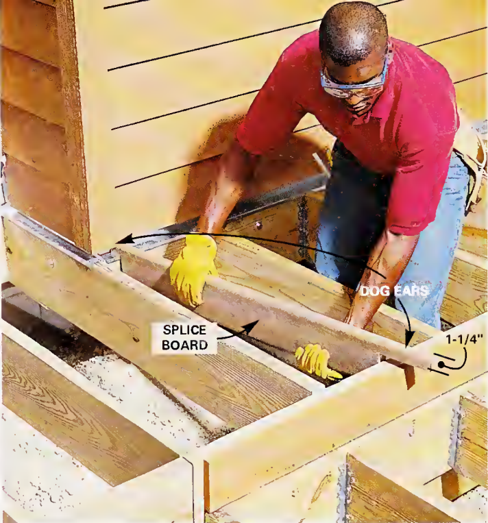
18 Cut notches in a piece of decking so that it protrudes above the joists 1-1/4 in. (flush with the top of the decking), away from the deck edge and even with the decking overhang.
