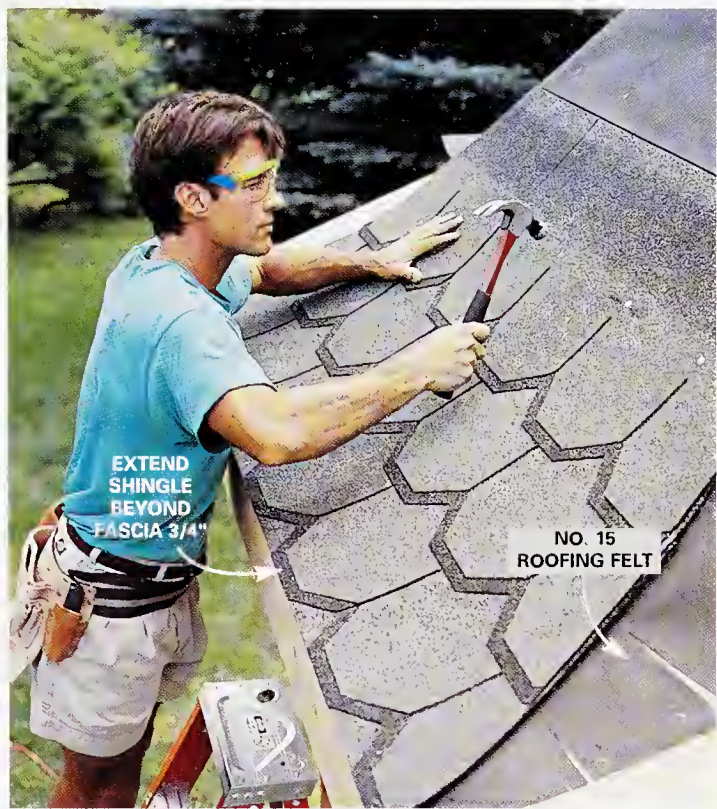
17 Shingle each lower roof section, then move to the opposite side. Keep the exposure consistent from side to side by measuring as you go.
