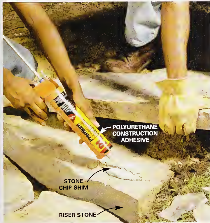
8 Shim unstable flagstone treads with stone chips. Tip the tread stone out of the way and glue the stone shims to the risers with polyurethane construction adhesive.
