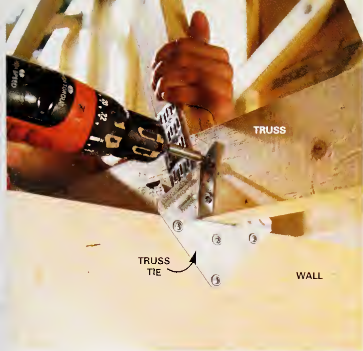
9 Screw truss clips to the tops of the walls and to the trusses with special 1-1/2 in. truss screws.
