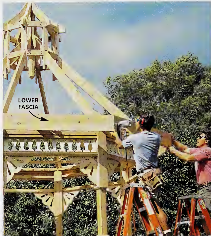
14 Nail the lower fascia (R1) to the rafter tail ends. Miter the ends with the saw set at 22-1/2 degrees.
