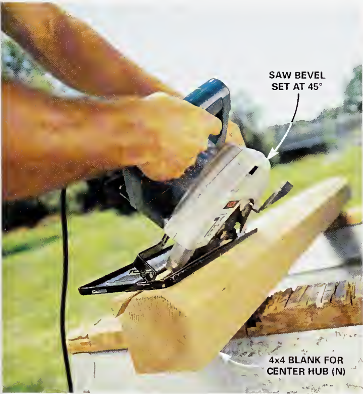
9 Shape the center hub (N) into an octagon. Measure in from each side about 1 in. and cut along this line with your saw bevel set at a 45-degree angle. The finished octagon should be about 1-1/2 in. on a side.
