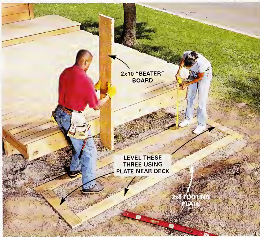
20 Dig trenches 6 in. deep and 12 in. wide and fill with gravel. Measure down from the deck to keep gravel levels within 1/2 in. of desired height. Lay down .60 foundation-grade lumber for footing plates a few inches longer than the intended planter length and width. To set the footing plates, measure down from the deck and pound on them with a heavy board. Use a 4-ft. level, working off the first plate when setting the plates that don't adjoin the deck.
