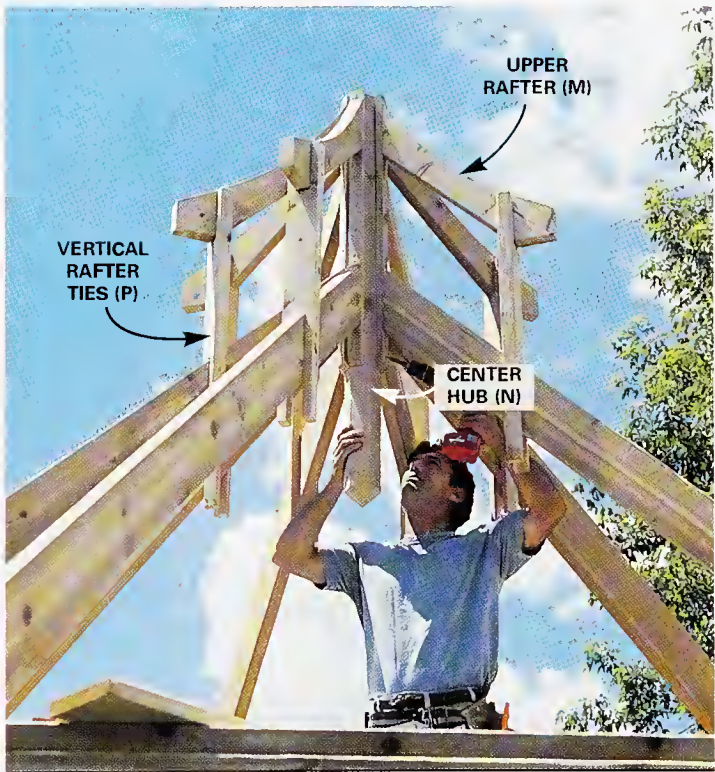
12 Fasten each rafter system to the center octagonal hub. Install opposite sides one after the other to maintain the shape of the octagon.
