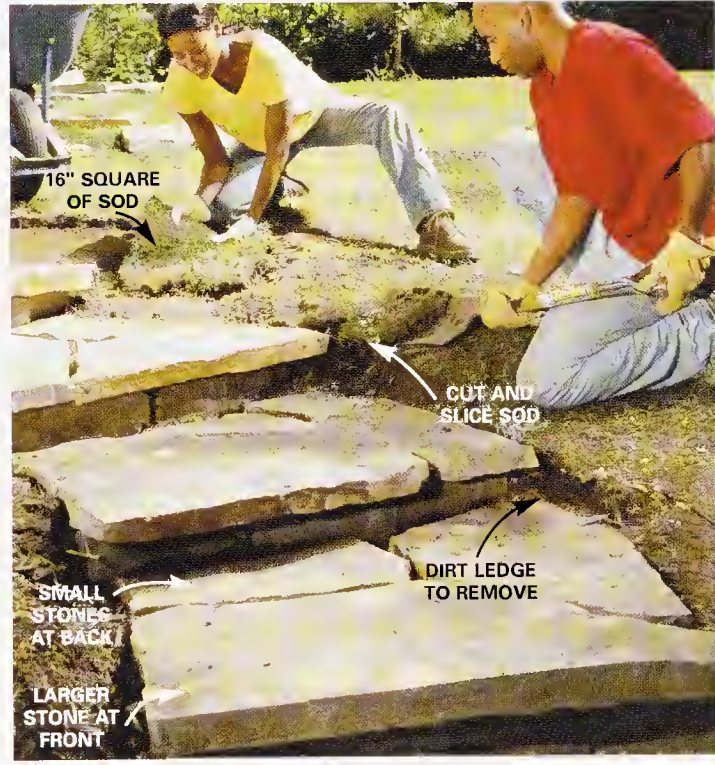
9 Cut 16-in. squares of sod from alongside the steps with a flat-blade shovel and lift them out. Remove enough soil to slope and blend the surrounding yard into the new steps. Replace the sod and water it.
