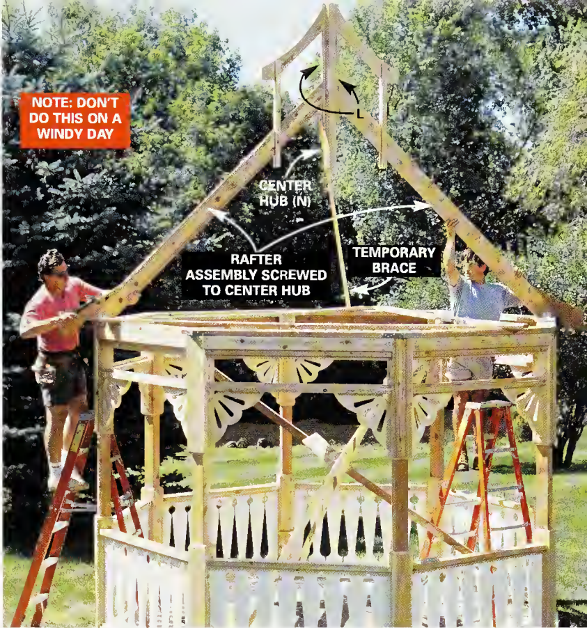
10 Attach two opposite rafters to the center hub. Then grab a partner and carefully walk the assembly up to position. See Photo 11 for nailing detail.
