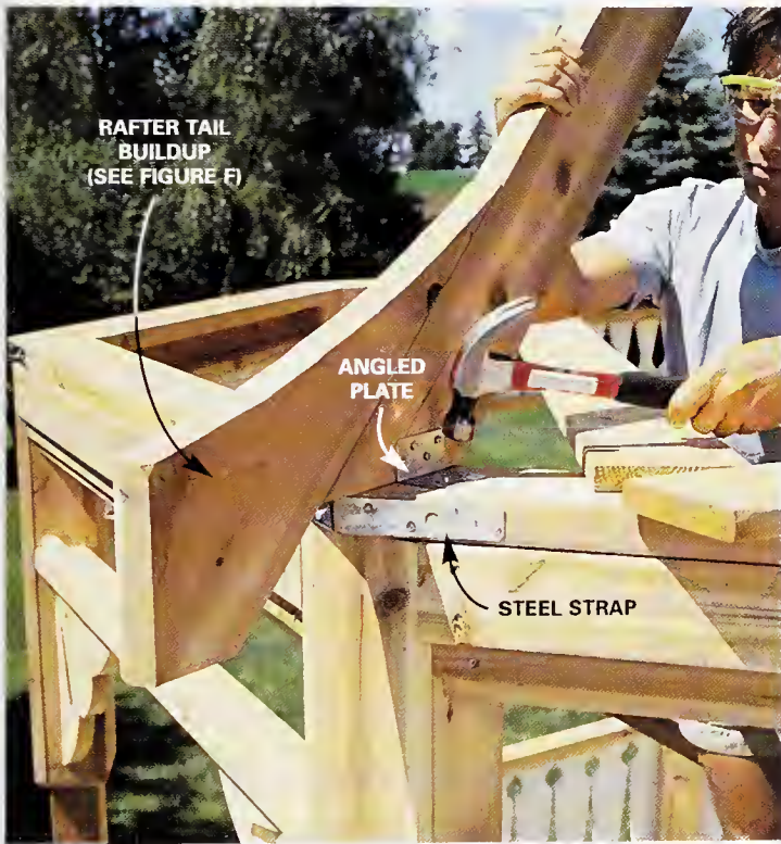
11 Nail the angled plates (see Resources, p. 252) to the rafter and to the top plates to secure the rafters to the structure.
