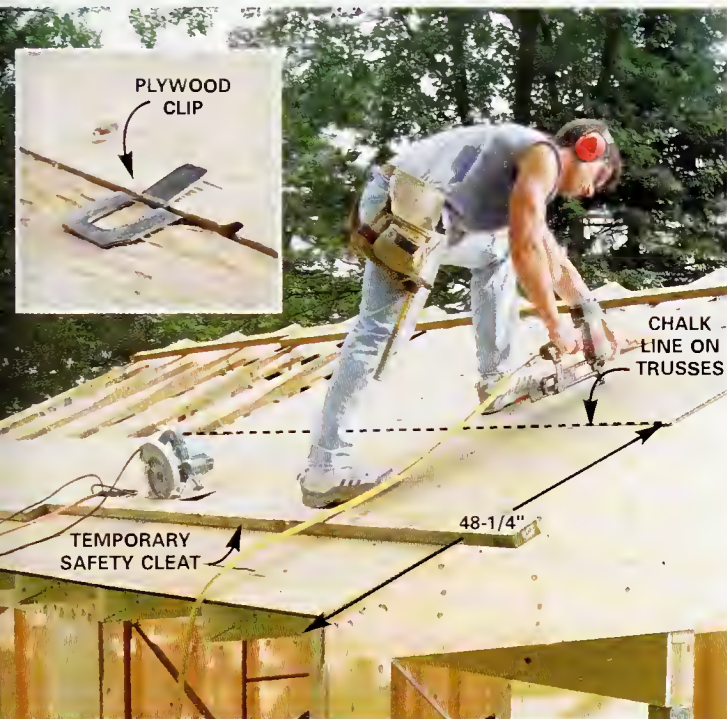
11 Snap a chalk line 48-1/4 in. up from the truss ends and nail down the first row of plywood sheathing. Add plywood clips midway between trusses and nail on the second row of sheathing.
