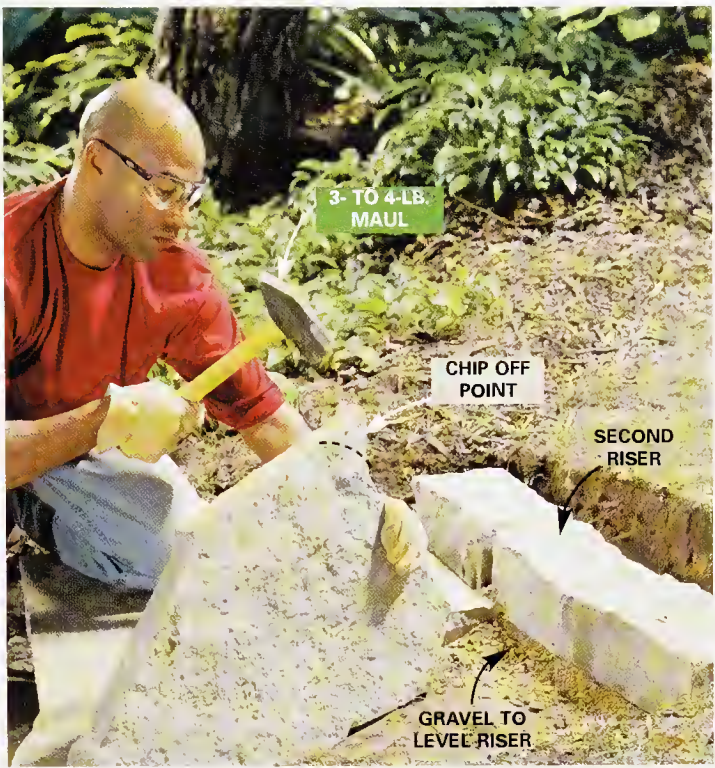
7 Trim stones for a better fit by chipping away at protruding pieces with a heavy maul. Wear safety glasses.
