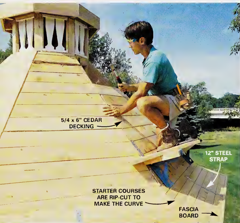
15 Nail the roof decking to the rafters with 8d nails. Be sure to screw (use 3/4-in. screws) the steel strap to the lower roof boards for extra support. The strap ties the narrower boards together to prevent sagging.
