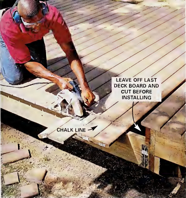
17 Cut off the excess decking. Measure the final cut lengths of the deck boards and cut the last deck board to length, rip it to width if necessary, and install it.
