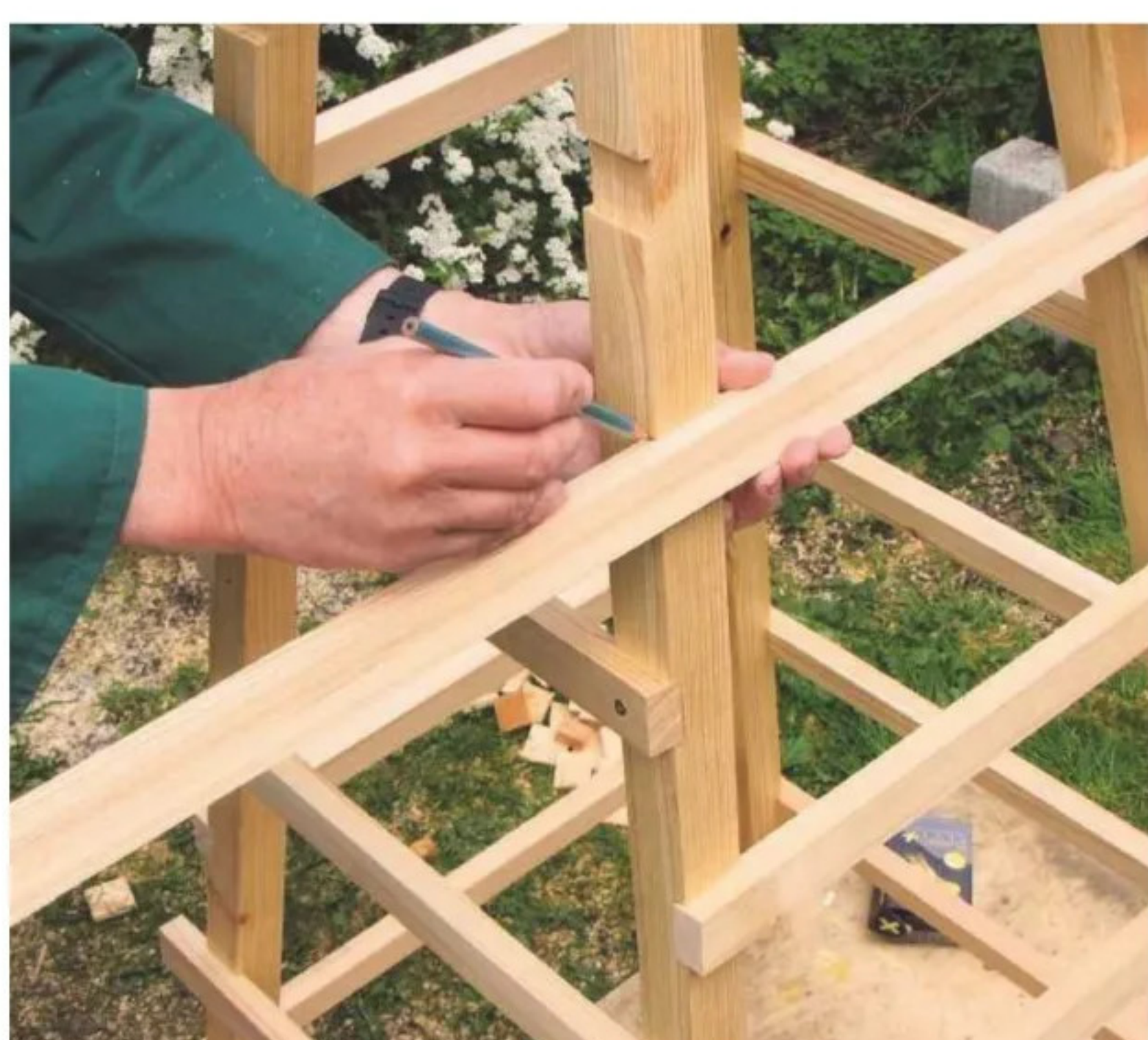
14 Once two opposite frames are assembled, join them together with the remaining rails
