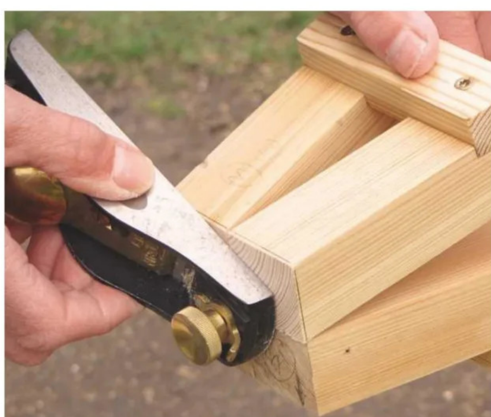
17 Trim upper ends of the legs level if necessary, taking care not to split the wood
