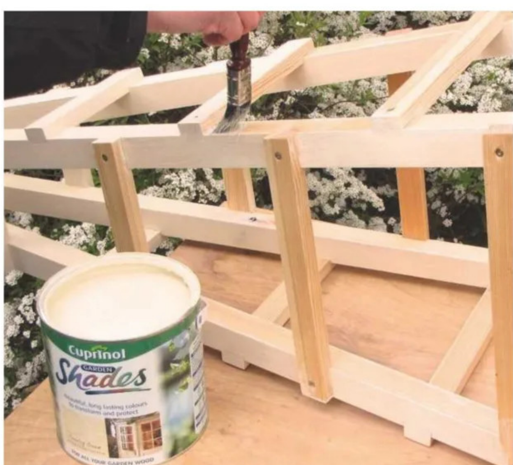
18 Brush on two coats of a suitable exterior paint, such as Cuprinol Shades – spraying is much quicker!
