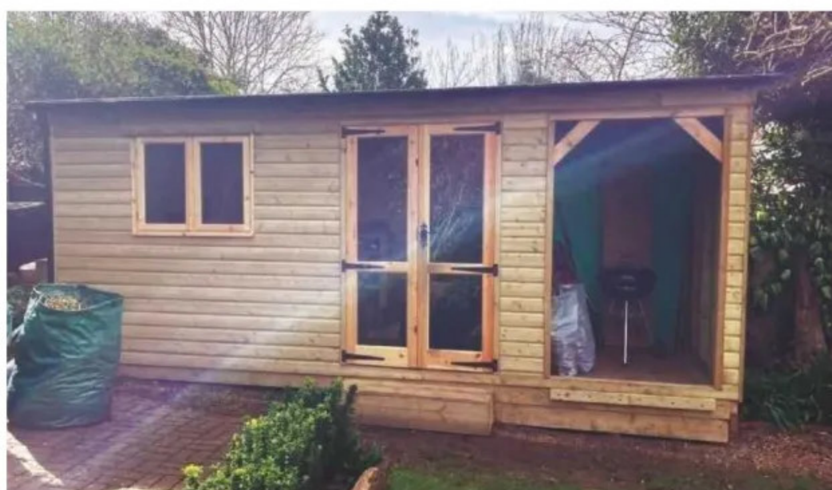
The newly-built garden workshop and bike store
