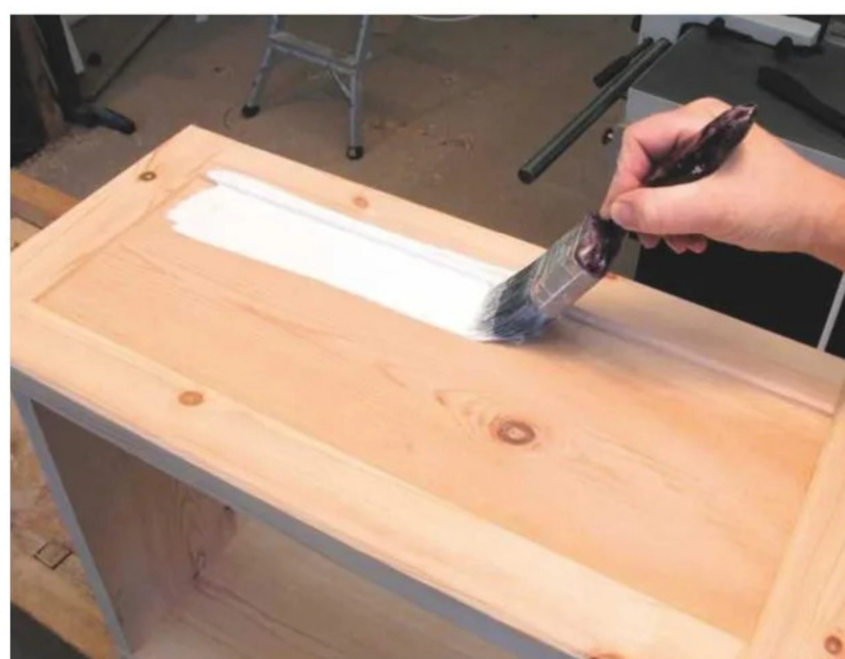
9 Primer paint applied to bare wood soaks into the surface and provides a firm key for later coats
