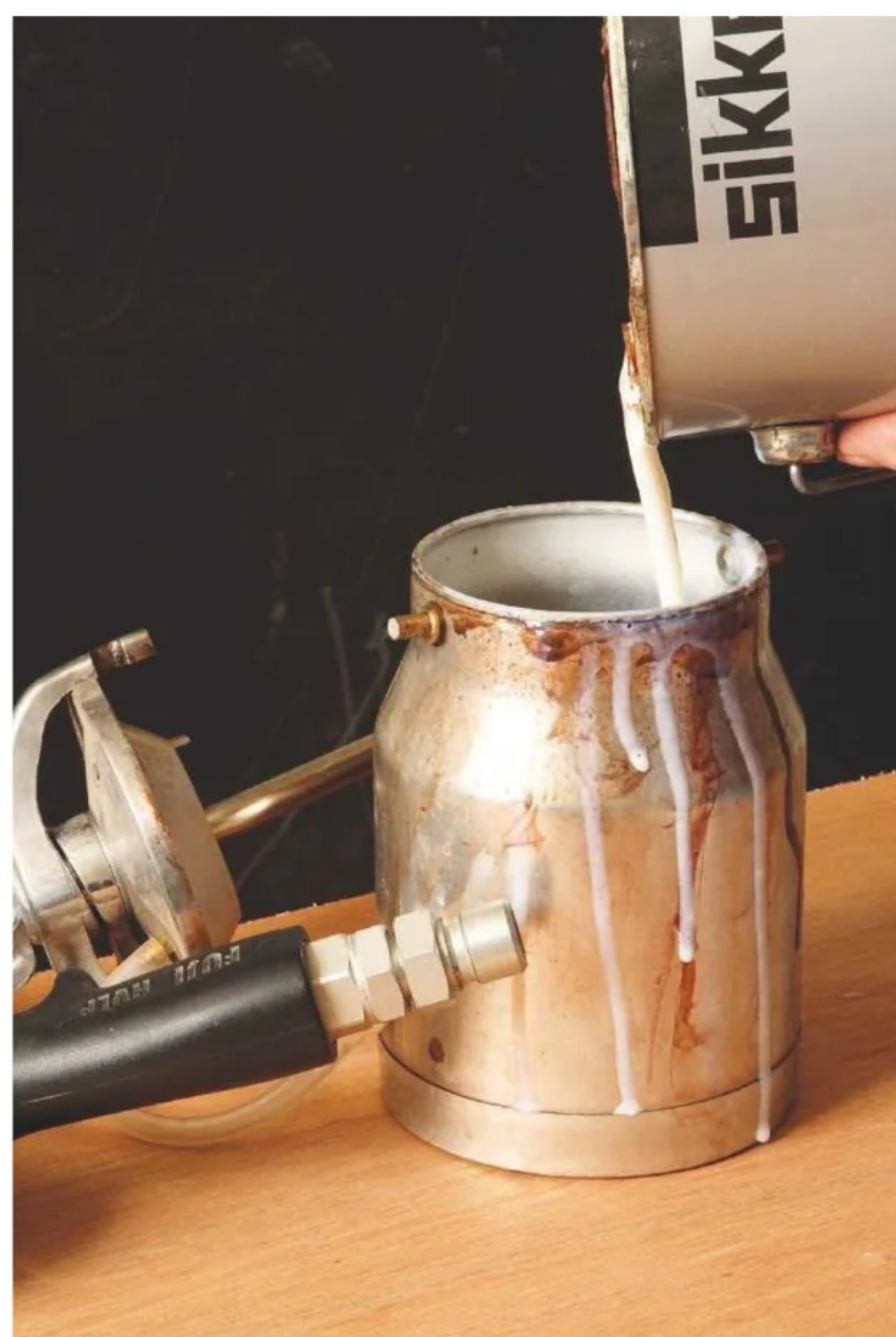
22 Spraying with water-based finishes is much less hazardous than traditional solvent-based spraying
