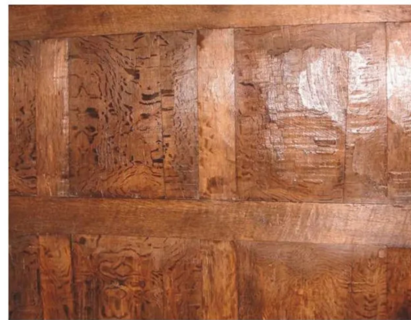
13 Beeswax applied to oak over centuries produces a deep lustrous patina, as seen on these Elizabethan wainscot panels
