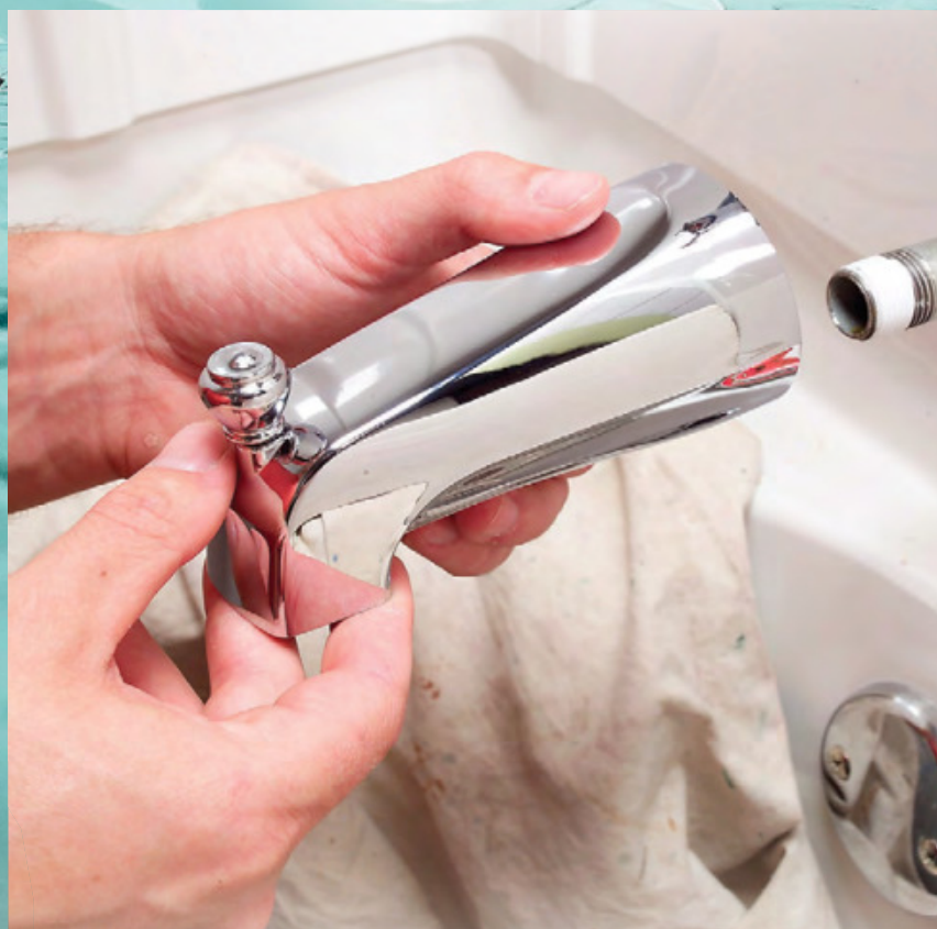
2 Wrap both ends of the new nipple with thread tape and screw it into the fitting inside the wall. Seal around it with silicone caulk and screw on the new spout.
