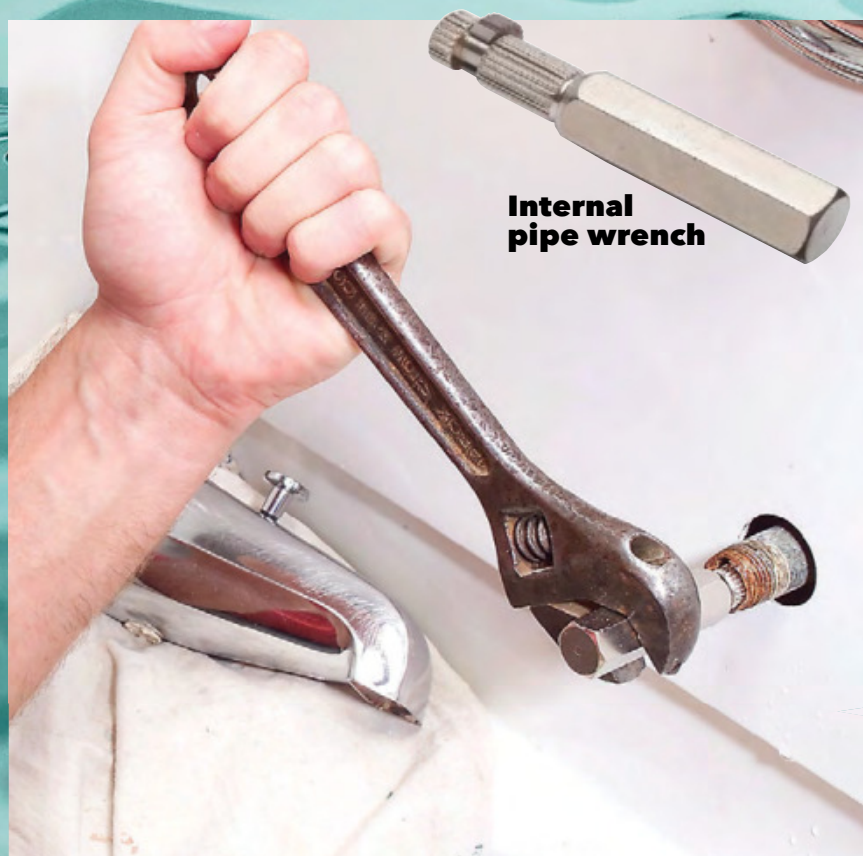
1 Unscrew the old nipple with a pipe wrench. If the nipple is too short to grab with a wrench, use an "internal" pipe wrench ($12).
