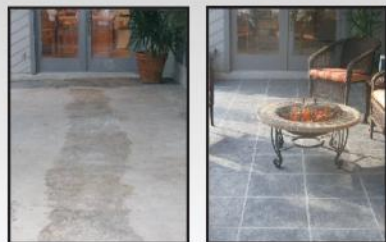
STENCILING BEFORE AND AFTER
