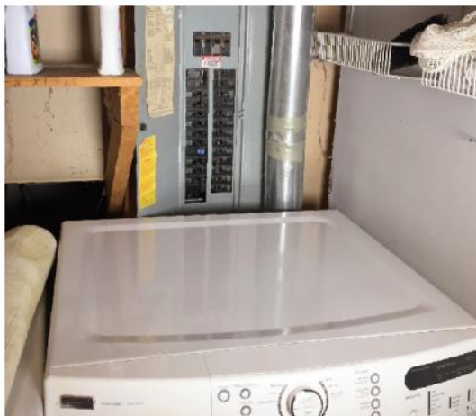
MINIMUM ACCESS CLEARANCE AROUND A SERVICE PANEL
