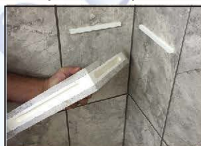
Silicone back and fill grooves
