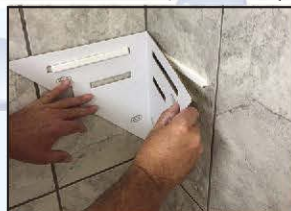
Glue on rails in slots
