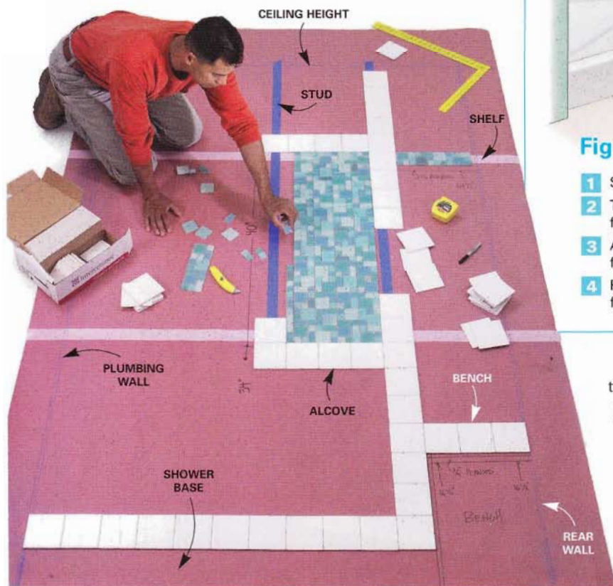
1 Plan the framing and tile layout for each wall on rosin paper cut to match the size of each wall.
