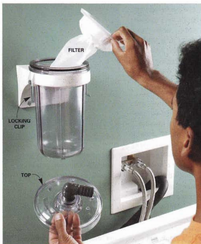
1 Set the mesh filter into the filter container and lock the top down with the locking clips.
