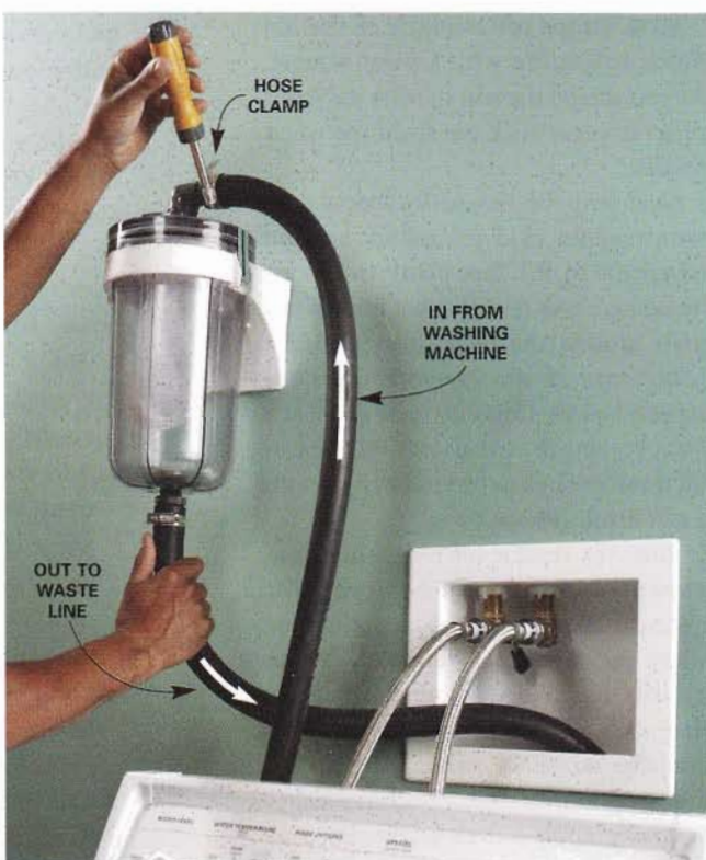
2 Screw adapters to the top and bottom of the filter. Push the discharge hoses onto the barbed fittings and tighten the hose clamps.
