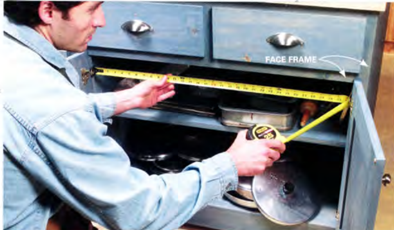
1 Open the cabinet doors to their widest point and measure the narrowest part of the cabinet opening (usually at the hinges).
