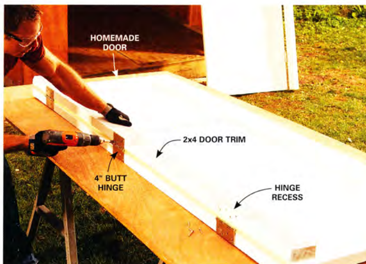
8 Hinge the doors to the side casings first. That way you can align the two doors easily and attach them by screwing the side casing to the shed.
