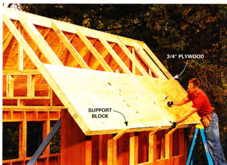
7 Nail blocks to the subfascia to support the plywood roof sheathing while you nail it on.
