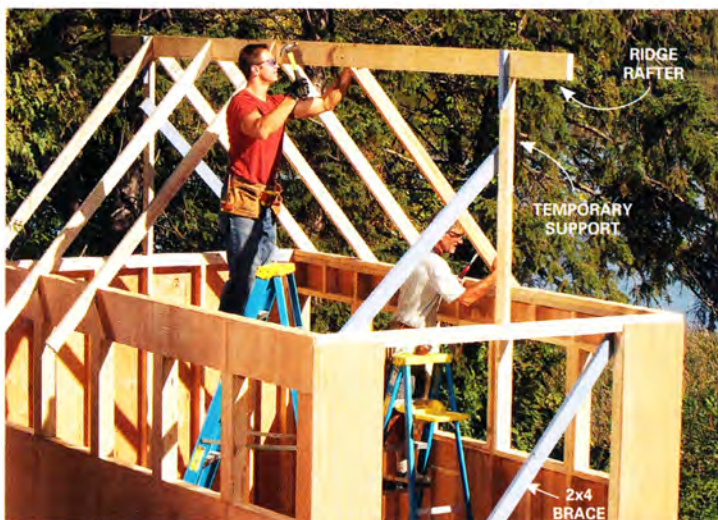
5 Position the ridge on temporary posts. Installing rafters is a lot easier if you have a helper at the other end.
