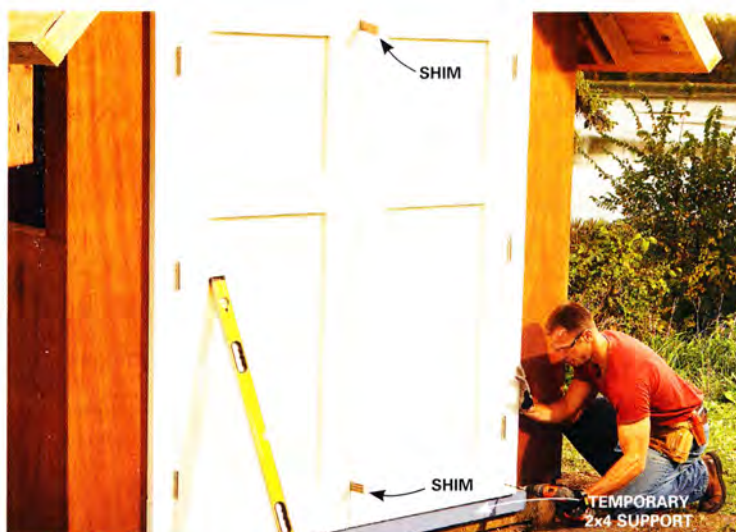
9 Position the doors with a temporary ledger and shims. Then screw the side casings to the shed for a perfect fit.
