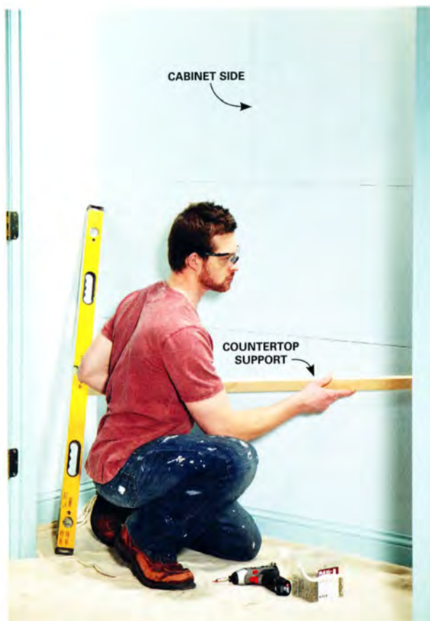
Figure B Drawer and countertop construction
