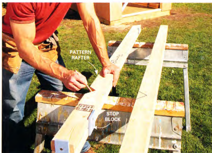
4 Cut one rafter and use it as a pattern to mark the others. Plywood stop blocks hold the pattern in position while you mark.
