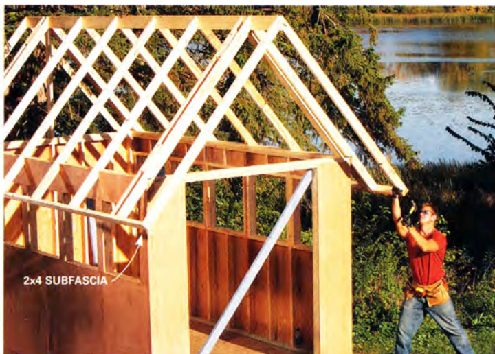
6 Add the subfascia before you install the outermost rafters. The subfascia supports the outermost rafters and allows you to drive shims behind it to create a perfectly straight nailing surface for the fascia board.
