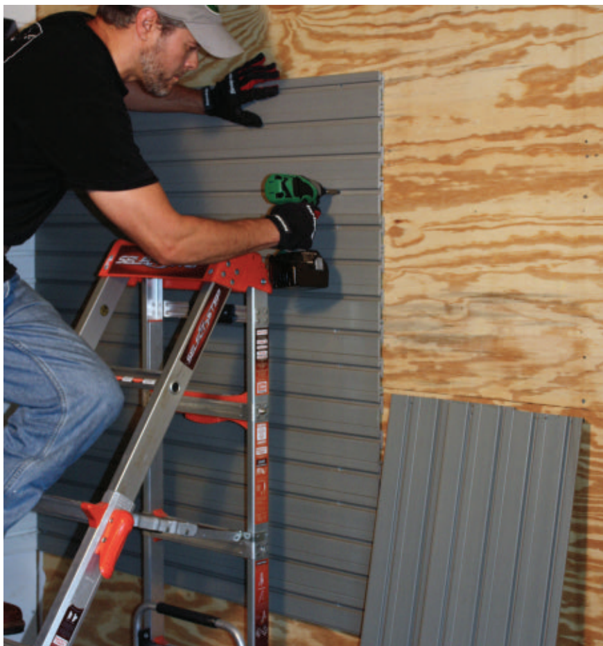
A slat-wall system requires the installation of 1/4" plywood over the wall studs to avoid deflection in the panels.
