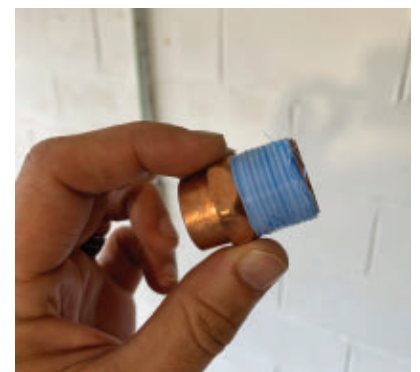
The filters tie into the supply line using threaded connections.
