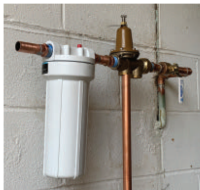
Next, we installed a pressure regulator and the sediment filter. The vertical tube pictured is a temporary support piece to carry the weight of the filter and regulator until the supply line has been completed.
