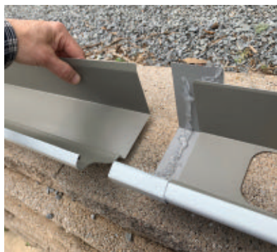
Gutter sections and downspout pieces are joined with 3-in. seamer pieces that are glued in place with gutter sealant.
