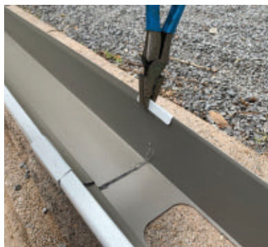
After they've been wrapped over the joint, the seamers hook over the front and back edges of the gutter, where they get crimped into place with pliers.
