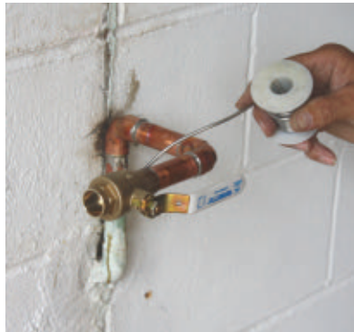
The filter location required installation of a new shut-off valve.
