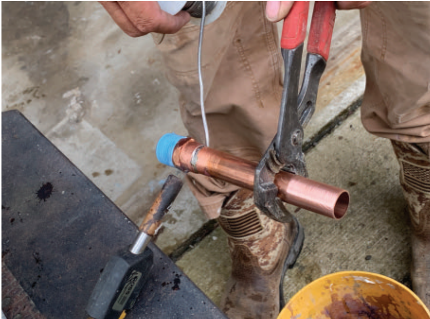
We installed the filters using soldered copper to ensure the connections maintained strength and rigidity over time.
