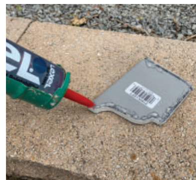
End caps get caulked with sealant and attached to the gutter end with a push-fit connection.
