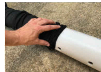
Apply the pipe sock.
