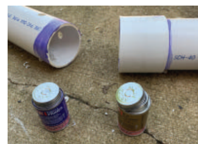
Join pipe lengths with PVC primer and cement.
