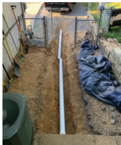
Testing the length of the pipe. This photo shows the scope of the project.
