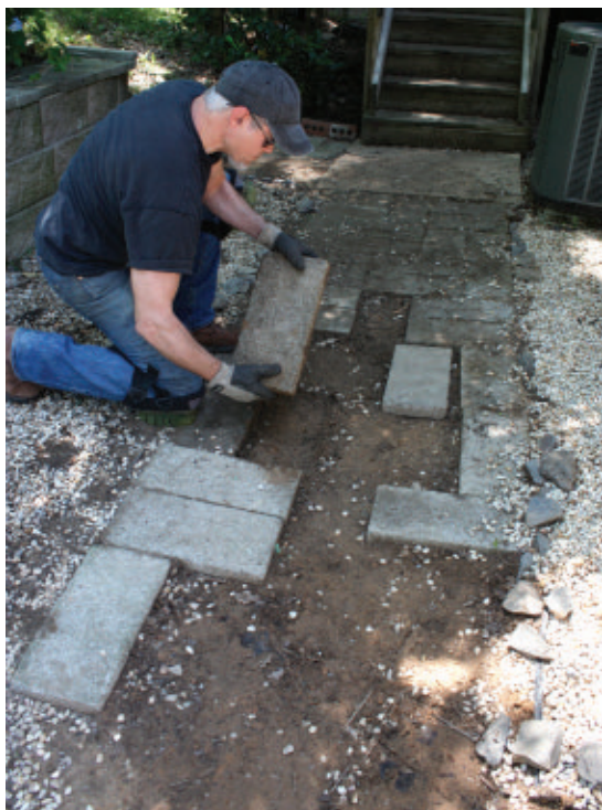
The problem area was covered by concrete pavers and pea gravel.
