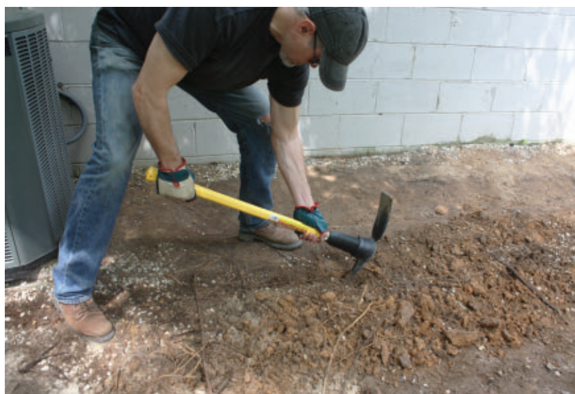
Use a mattock to break ground. Allow the weight and sharpness of the tool to do the work—there's no need to take big swings.
