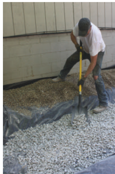
The drain trench was recessed into a broader trench I dug for the paver walkway, which I filled with gravel, compacted and leveled.
