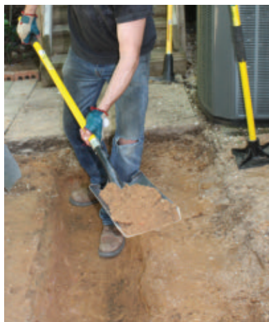
Shape the trench with shovels.
