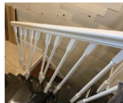
The balusters remained attached to the rail, and the whole assembly was lifted out as a single piece.
