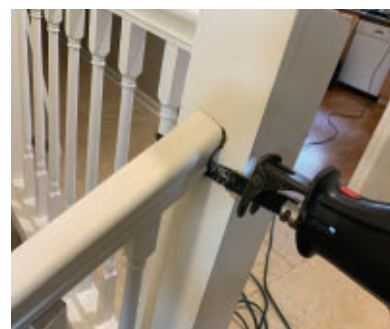
We used a reciprocating saw to cut the old rail off the existing newel.
