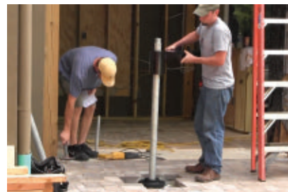
Assembly of the Arke kit begins with installation of the base-plate and the center pole.
