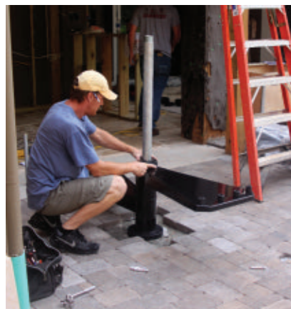
The treads and spacers slide over the pole.
