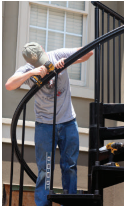
The handrail screws on one section at a time.
