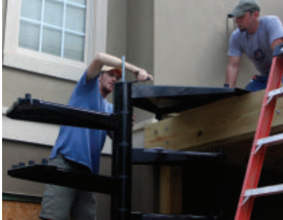
The staircase shown has a mezzanine landing.
