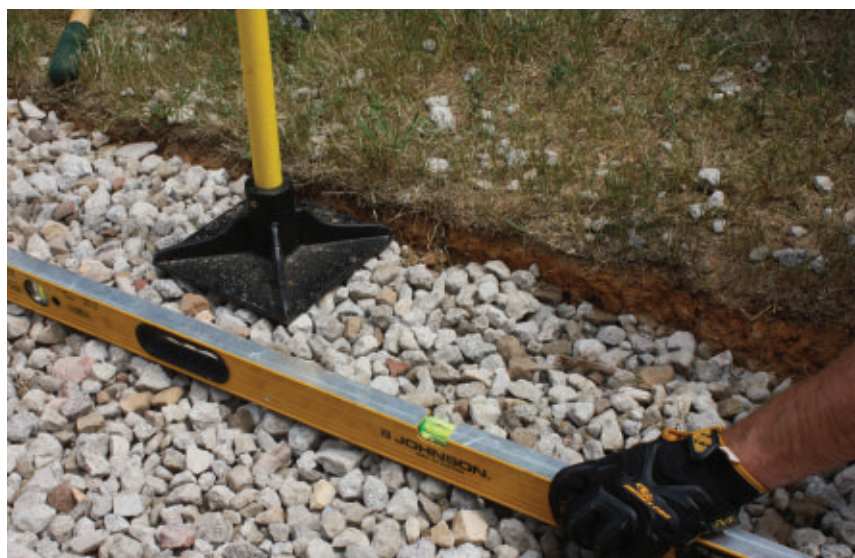
Tamp down and level the gravel bed.
