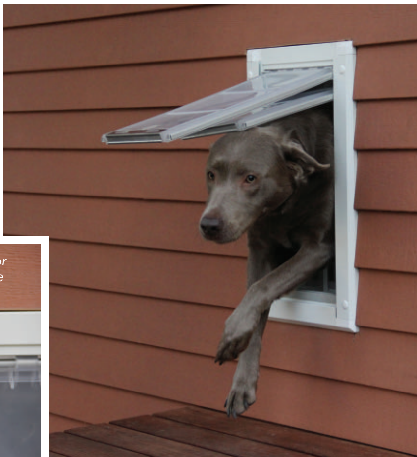
We used an oscillating multi-tool to carefully cut the siding to recess the door into the wall, giving it a more finished appearance and eliminating air gaps.
