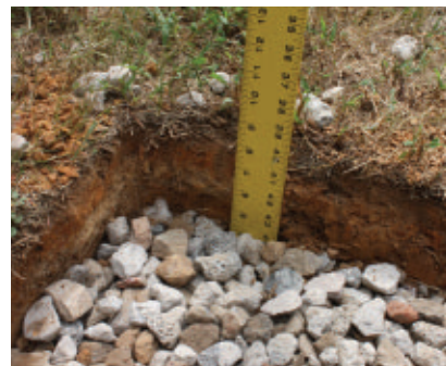
Dig deep enough to account for the gravel base (4" after compaction) and concrete pour (4").
