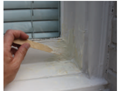
The PL FIX product can be cut and shaped to match existing wood profiles.
