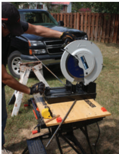
I used a cutoff saw to trim the rebar to size for the reinforcement grid.
