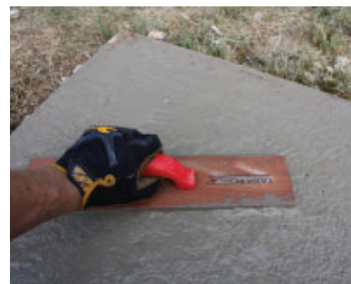
Float the surface of the slab to bring the cream to the top.
