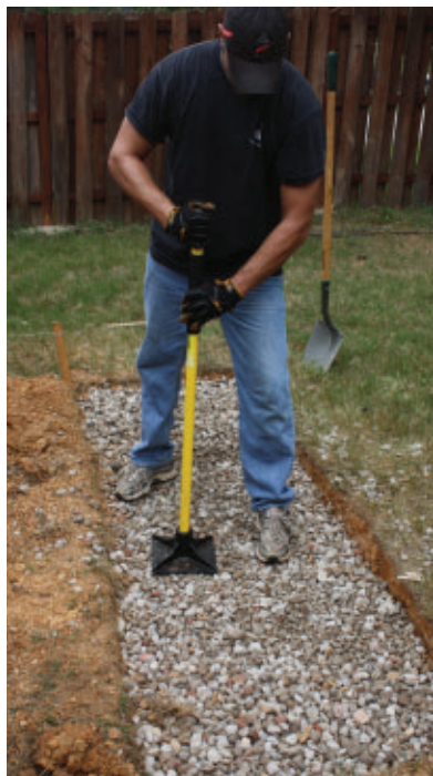
Add a gravel base for the slab.
