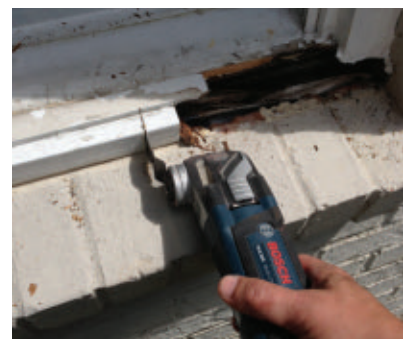
An oscillating multi-tool like this Bosch Multi-X is a great gadget for cutting out damaged wood.
