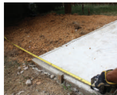
After the concrete fully cures, it's ready for use as a walkway or footing.
