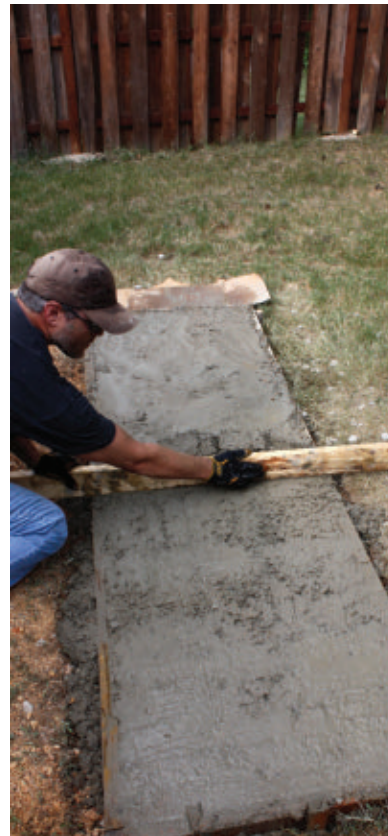
Screed the concrete even with the form.
