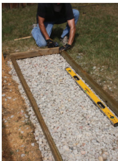
The concrete form was made from treated 2x4s.
