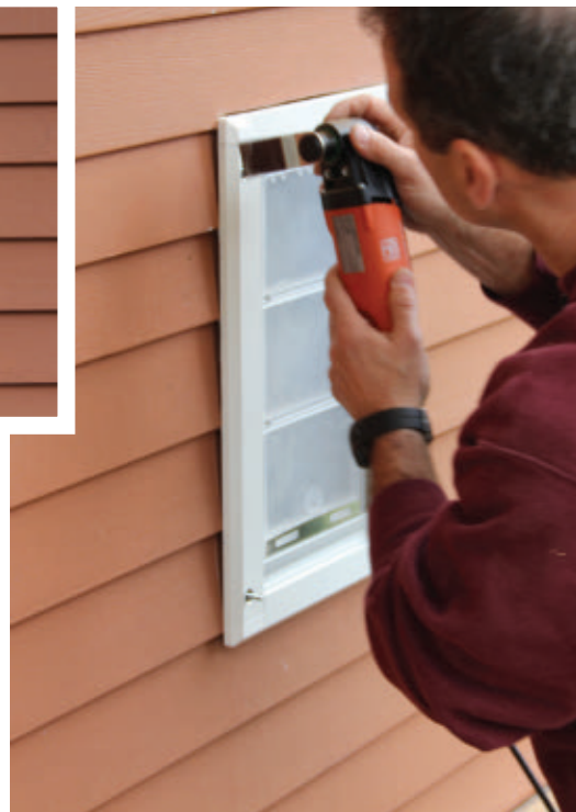
We used an oscillating multi-tool to carefully cut the siding to recess the door into the wall, giving it a more finished appearance and eliminating air gaps.
