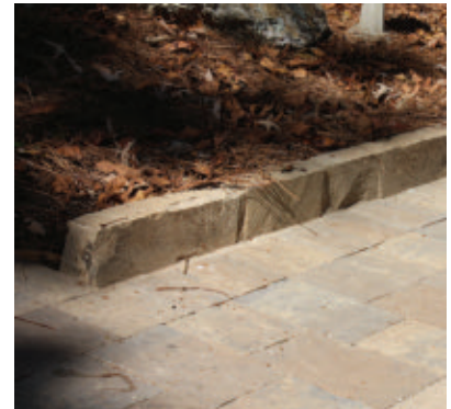
The uphill side of the patio was lined with tall edging bricks to divert runoff from the patio surface.
