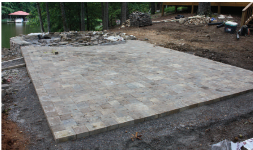
The exposed edges of the pavers will be buried by substantial landscaping so the patio surface will be just above ground level.
