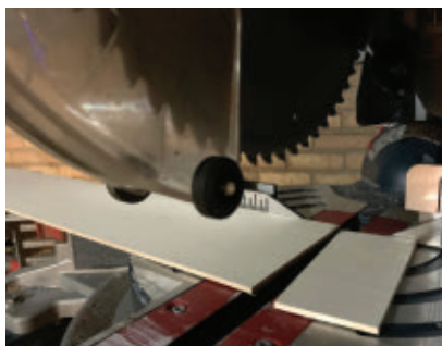
A miter saw is handy tool for making quick cuts in the planks.
