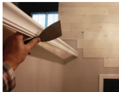
When removing trimwork, pry it off carefully and pull out the nails if you have any intention of reusing the material.
