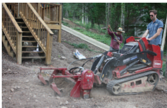
Site prep of this large patio requires removal of dirt, stone and rocks. A skid-steer with a power rake attachment breaks up the earth.
