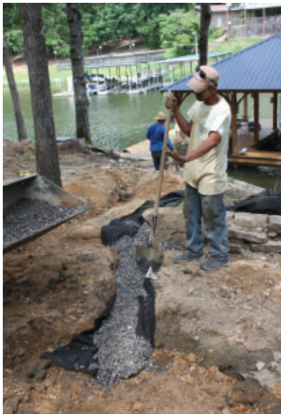
Site conditions and patio design will determine how to manage drainage. This patio included a circular fire pit with a drainage trench, which was lined with landscape fabric and filled with gravel.
