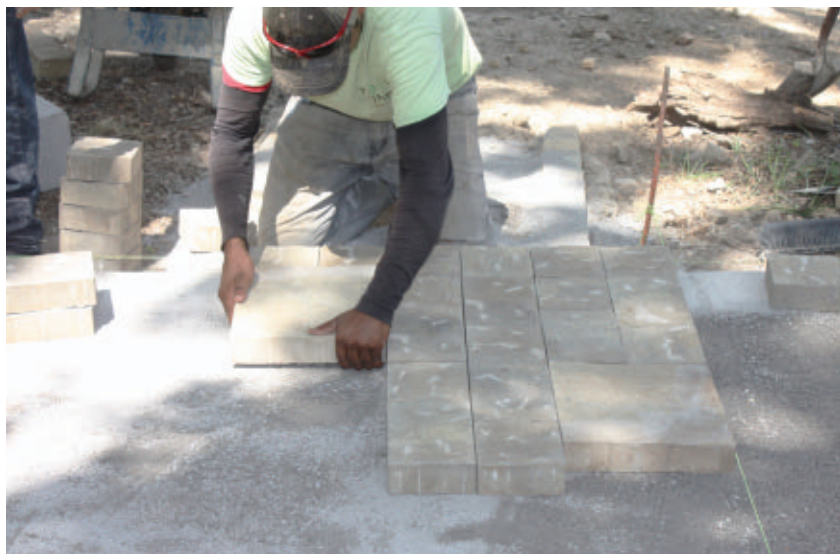
The choice of brick pattern can minimize cutting of the pavers.
