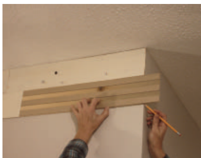
Carefully mark the face of the planks for cutting.
