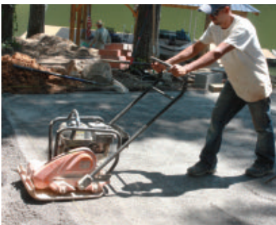
A vibratory plate compactor will be used in multiple phases of construction.
