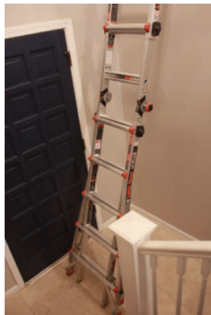
All remodeling jobs are different so plan the project in advance. This one required a telescoping ladder to access the tall walls above a staircase.
