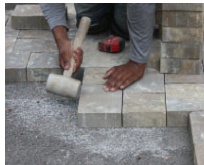
A rubber mallet should be used to set the pavers into the base.
