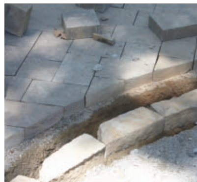
The fire pit was surrounded by the circular edge of the patio, which had to be cut at an arc.
