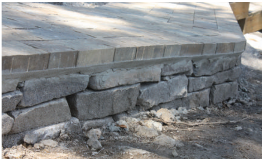
To accommodate the slope, a drystack stone wall was built to support the downhill side of the walkway, and the edge pavers were mortared onto the wall as the top course.
