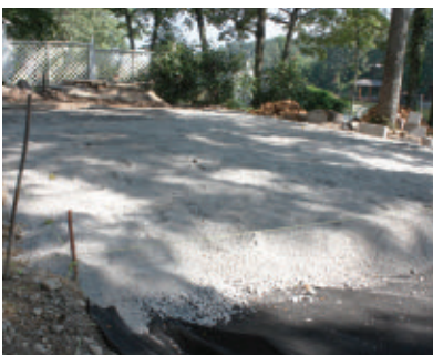
The bed of crushed rock should be spread evenly over the patio site and thoroughly compacted.
