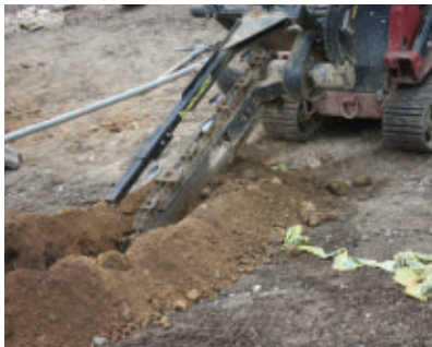
A trencher attachment digs the ditch for an electrical line as well as a drainage trough for the fire pit.
