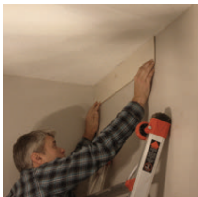
Begin the first row in a corner.
