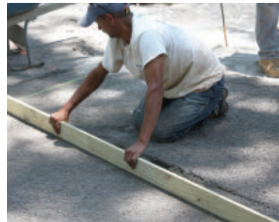
The bed of crushed rock should be screeded evenly in preparation for the paver surface.
