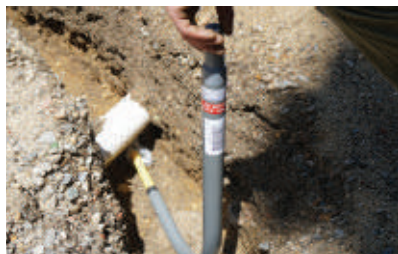
The gas line runs through the bottom of the fire bowl to connect with the burner.
