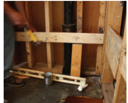
Wood stringers were installed over the studs.
