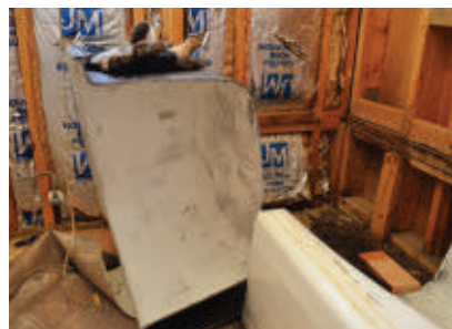
Next, a pry bar helped to pull the two halves away from the wall for disposal.
