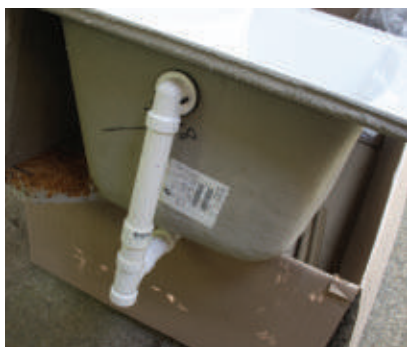
This photo shows the tub fitted with the universal PVC drain kit.
