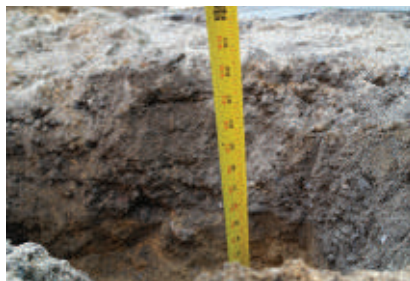
The gas line had to be buried in an 18" deep trench.
