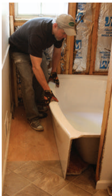
Dry-fit the tub to troubleshoot any issues prior to mixing the mortar.
