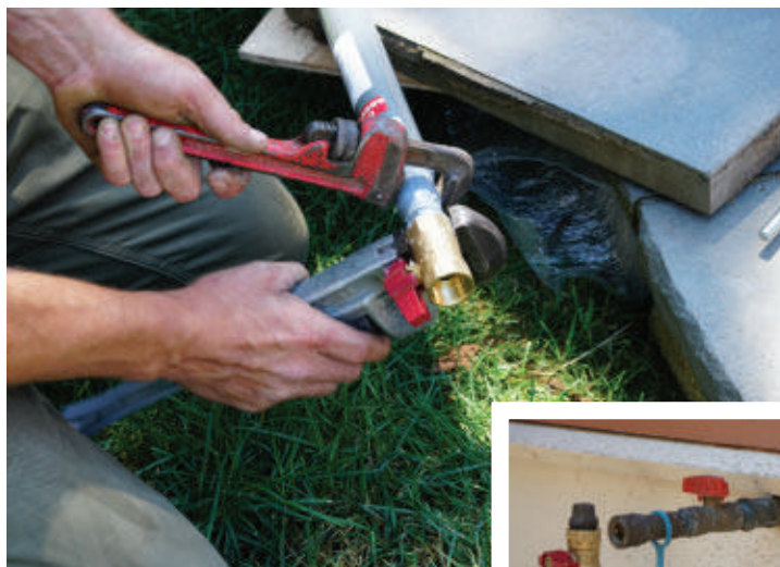
The rigid end sections were fitted to connect with the supply valve and the burner of the fire bowl.
