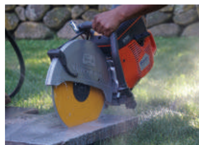
To cut the bluestone, the crew used a masonry saw. The blade should be kept wet when cutting to prevent it from warping and extend its usable life.
