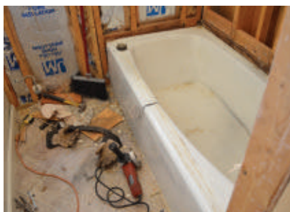
The wall sheathing was removed from around the old tub.
