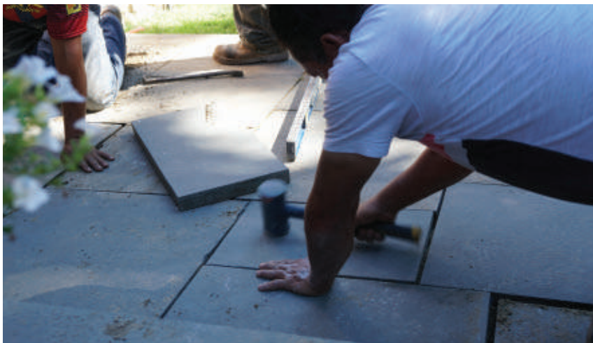
The subbase should be properly compacted and the bluestone pavers must be carefully replaced and set securely.
