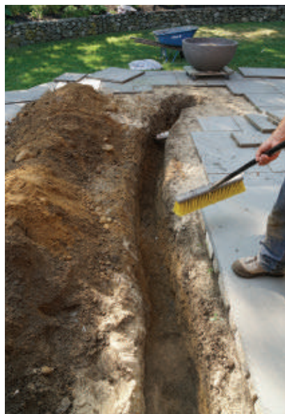
The fire bowl for this project is fueled by gas and required a new gas line installed beneath the patio.
