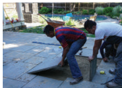
The patio had to be reconstructed after the fuel line was in place.
