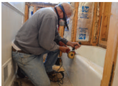
To remove the old tub, we used an electric grinder with a metal-cutting wheel to cut it in half.
