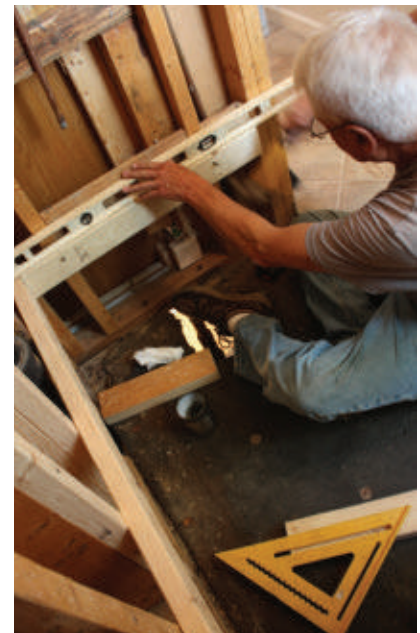
The stringers are intended to level and support the tub deck, but the rim must NOT support the weight of the tub.
