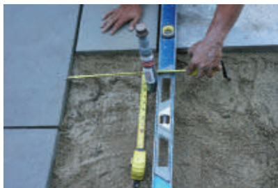
The crew had to map out the location of the gas pipe to cut access in the bluestone.
