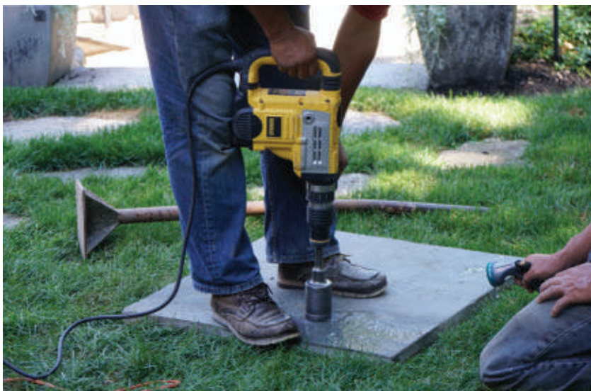
A masonry hole saw was used to drill access for the gas line. Water should be used to cool the cutting action.
