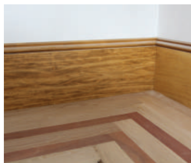
The ends of the intersecting rows of the border use a consistent and overlapping pattern in the corners, not unlike a herringbone pattern.
