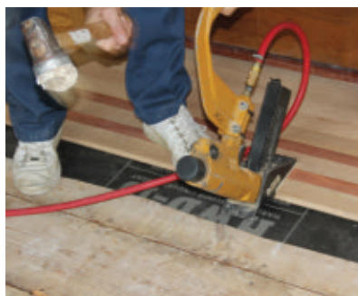
The flooring was fastened over a moisture barrier using a heavy-duty flooring stapler.
