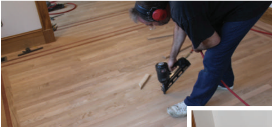
Face-nail to fasten the final row securely.
