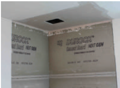
Complete the shower enclosure substrate from top to bottom.
