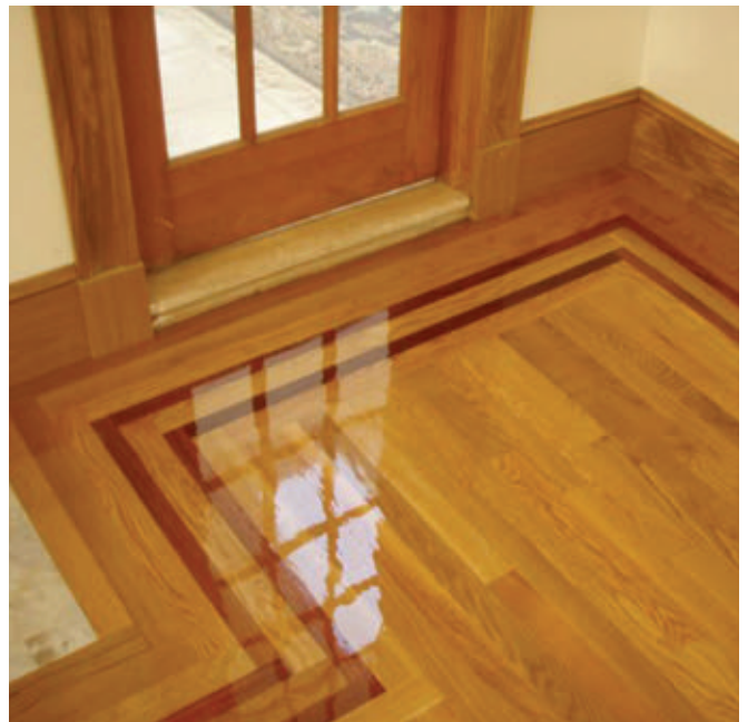
Shown is the completed floor after finish has been applied.
