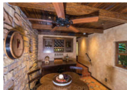
Tongue-and-groove planks with exposed woodgrain can give your ceiling a natural rustic appearance. Fasten the boards to plywood or furring strips.
