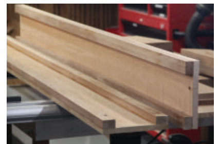
The door trim's side columns, plinth blocks and headpiece were all constructed with 1-in. return strips along the edges to conceal the plywood backboard that would be installed behind it.
