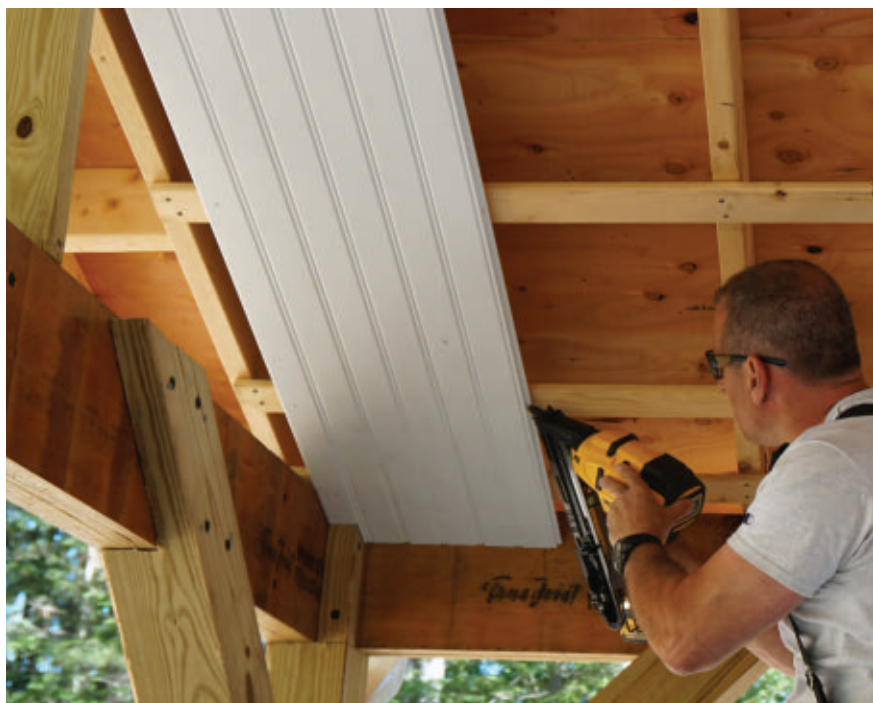
A similar option is a beadboard ceiling. You can conceal the fasteners of the boards nailed to the ceiling by blind-nailing inside the T&G joints.
