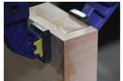
Returns were also installed in the ends of the headpiece.
