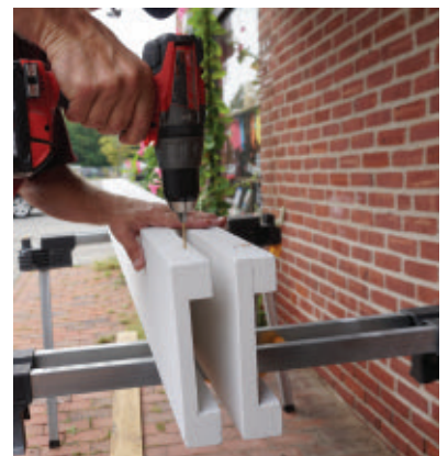
The cedar columns were predrilled before being fastened over the plywood backing.
