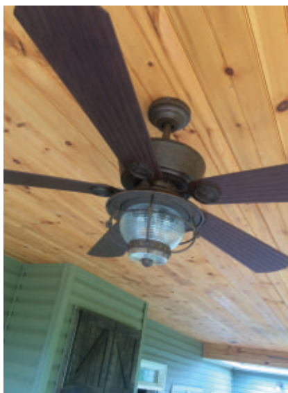
Tongue-and-groove planks with exposed woodgrain can give your ceiling a natural rustic appearance. Fasten the boards to plywood or furring strips.
