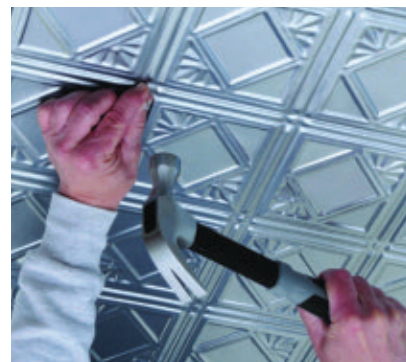
Metal ceiling tiles can be installed with cone-head nails that have a matching finish. Photo © Armstrong Ceilings.
