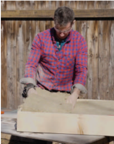
Frames filled with RockWool help slow the sound.
