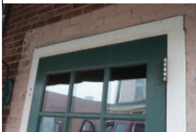
The owner wanted to conceal the pink paint that surrounded the door.
