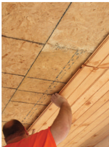
Tongue-and-groove planks with exposed woodgrain can give your ceiling a natural rustic appearance. Fasten the boards to plywood or furring strips.
