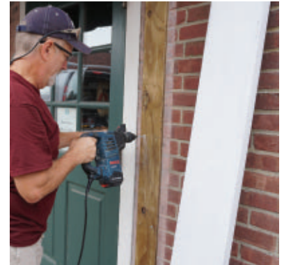
Before installing the columns, the plywood backer had to be fastened to the brick. The plywood required predrilling for the masonry anchors.
