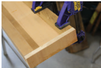
The need to conceal the paint gave us the width of the surround, so we made the trim pieces out of accordingly sized of cedar.
