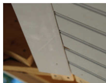
The boards intersect the temporary board at the top of the slope.
