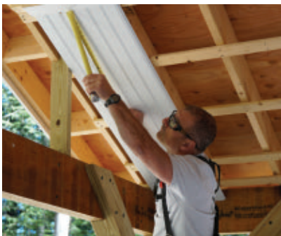
Measure the boards to make sure you're installing them parallel to the porch walls.
