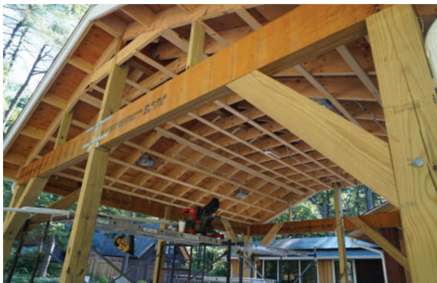
We first installed 1x3 strapping 16" on center over the ceiling rafters.
