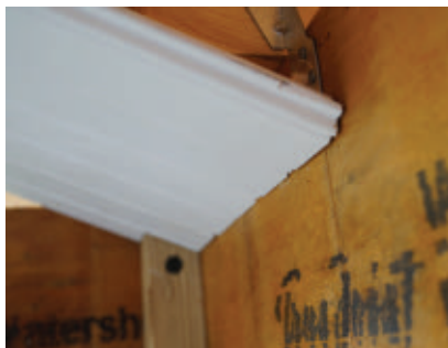
The boards terminate at the LVL band of the porch roof.
