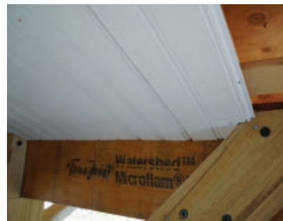
Here we had to cut room for the roof bracing.
