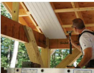
It may be necessary to tap the boards together to close the seams, but be careful not to damage the joint.
