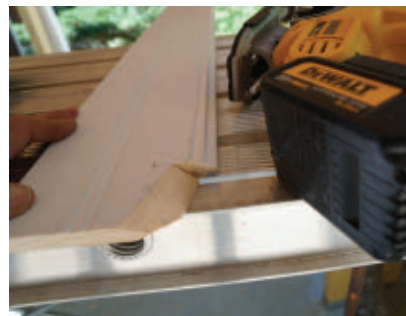
Use a jigsaw to notch boards to fit around obstructions.
