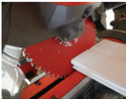
Cutting a bevel at the board ends will help ensure a snug fit.
