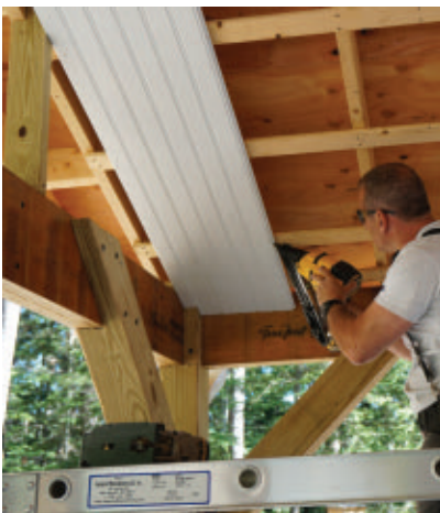
The tongue-and-groove beadboard boards are blind-nailed onto the nailers.
