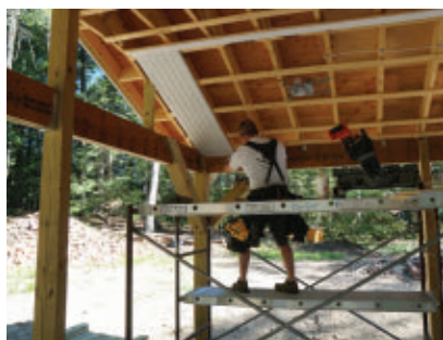
Multi-level scaffolding will make a job like this much easier.
