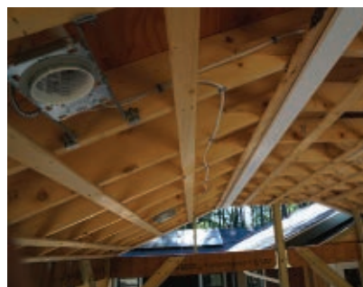
A temporary board at the top of the roof slope served as a guide for installing the beadboard boards.
