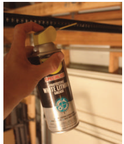
Use white lithium-grease to lubricate the chain and screw of an automatic garage door opener.
