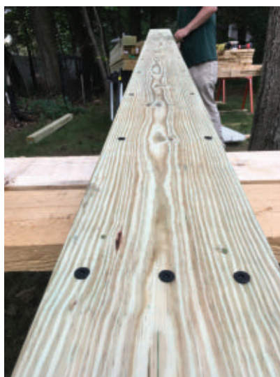
On this treehouse, the TABs supported beams made from doubled pressure-treated 2x10.
