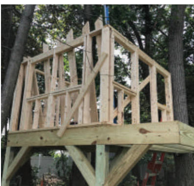
This particular treehouse was an 8x8' structure with two 36" decks on either end.
