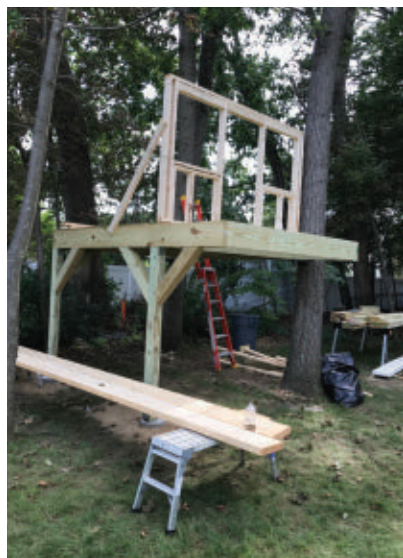
The remainder of the tree house is essentially a small shed built atop the platform.
