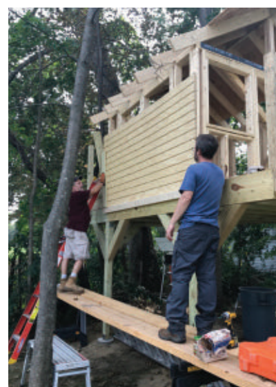
T1-11 siding oriented with horizontal lines provides a rustic clapboard look.
