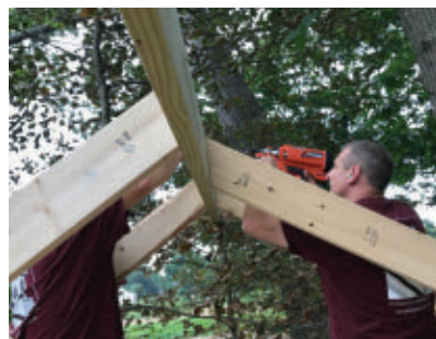
The roof rafters were made from 2x6 and reinforced with Simpson hurricane ties.
