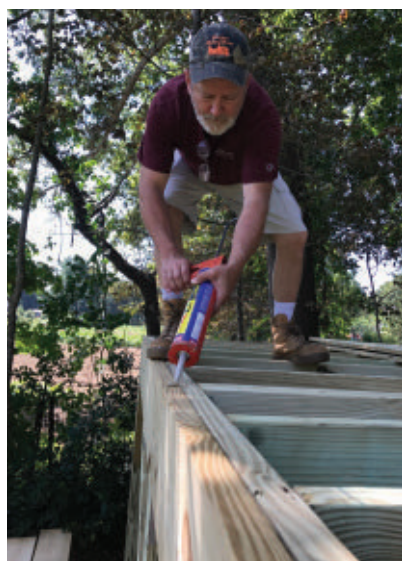
The decking of the treehouse is 3/4" CDX plywood glued and screwed to the joists.
