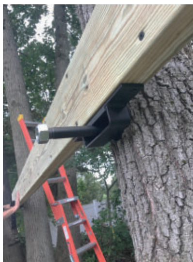
The brackets slide over the perch of the TABS.
