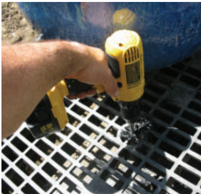
Next, I drilled a hole in the grate for the standpipe. Test-fit the standpipe.
