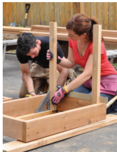
We used a framing square and a layout square to get the staves nice and square.
