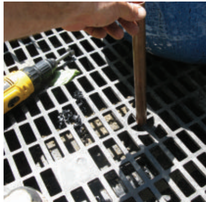
Next, I drilled a hole in the grate for the standpipe. Test-fit the standpipe.
