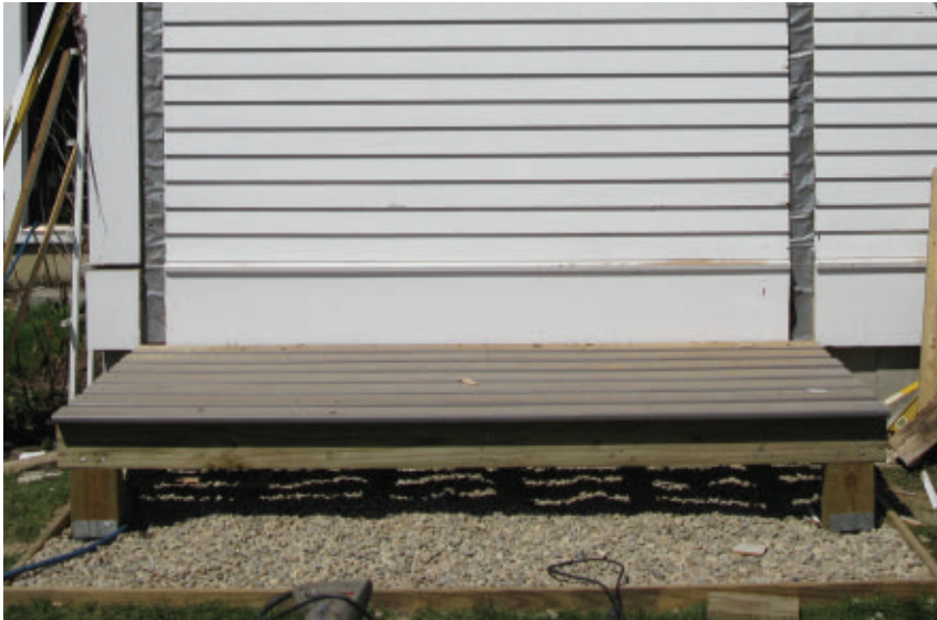
The floor boards were spaced to facilitate air flow to the firewood.
