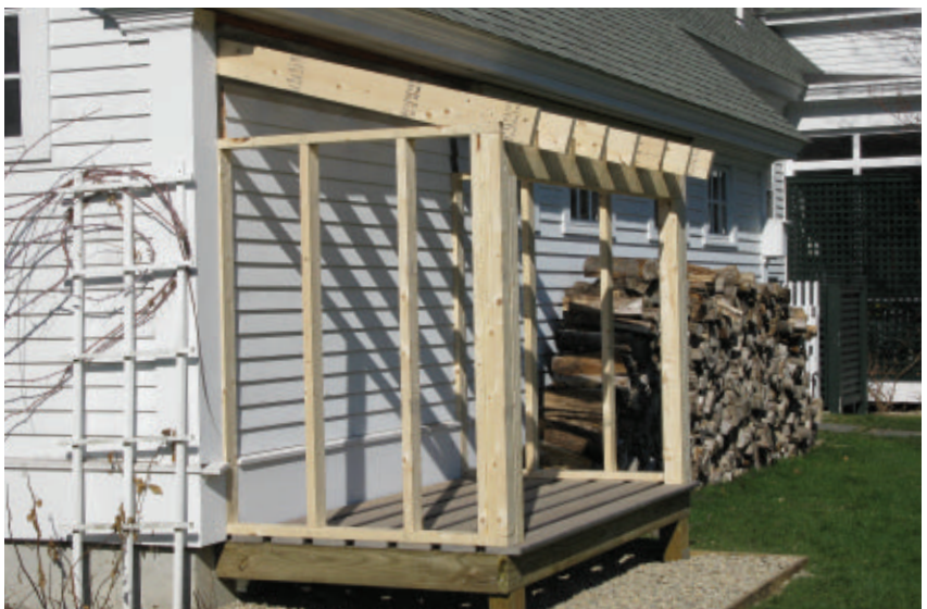
We laid out a 3- to 4-pitch roof and installed a header on the side wall of the garage.
