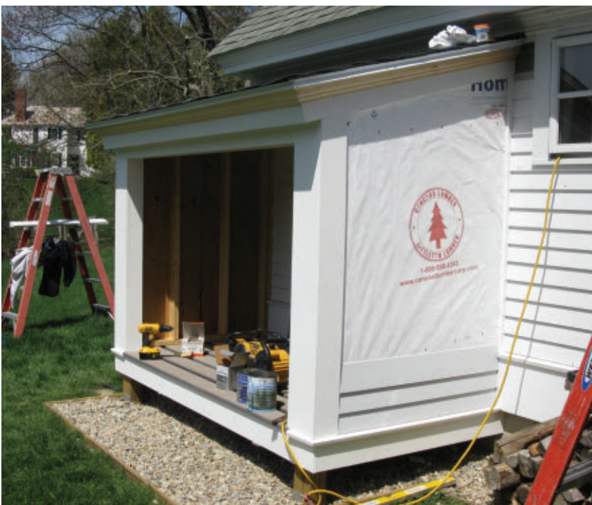
The walls were then sided with pre-primed Western Red Cedar clapboard.
