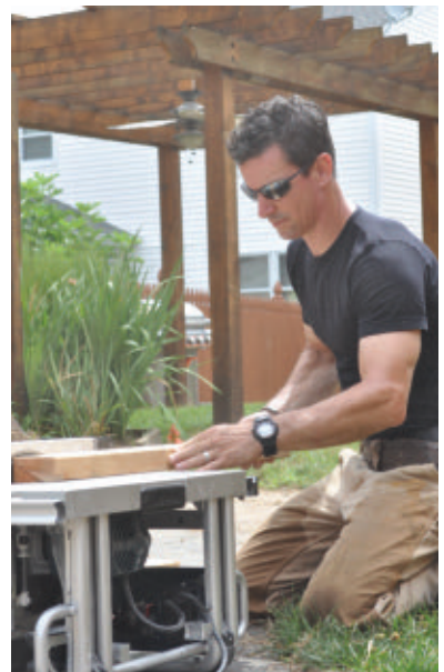
Staves are 2x6 ripped in half on the table saw.
