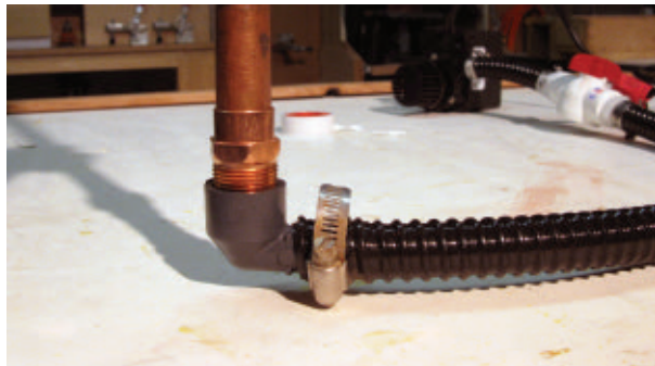
To make the transition from pump hose to main fountain, I used a 90-degree PVC irrigation elbow insert (1x3/4") to connect the copper pipe.
