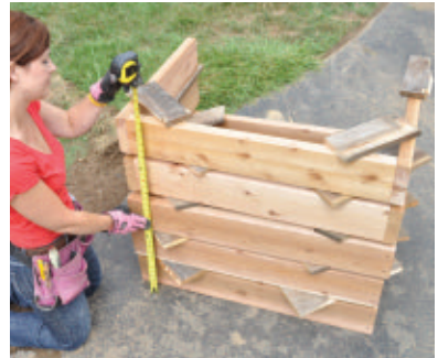
Use 1x scraps as spacers for uniform gaps that let air into the bin.
