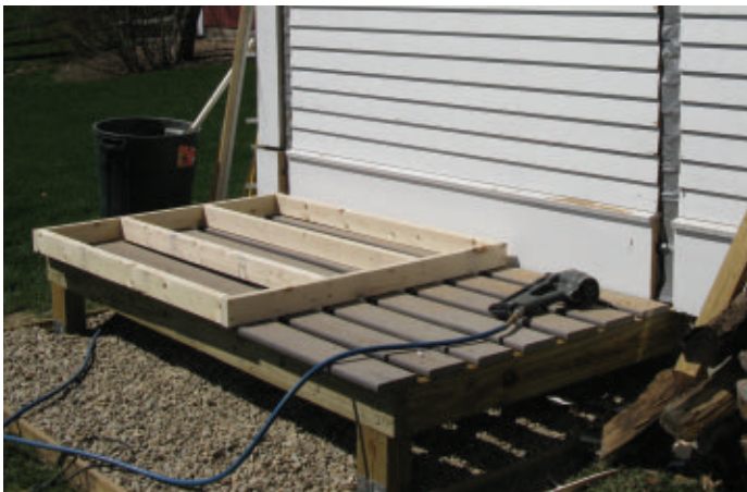
The floor boards were spaced to facilitate air flow to the firewood.
