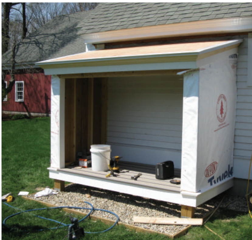
The sheathing was wrapped in building paper.
