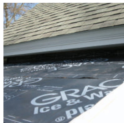
The roof sheathing was protected by Ice & Water Shield.
