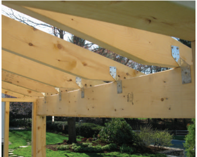
The 2x6 rafters were installed and additionally supported with rafter clips or "hurricane ties."
