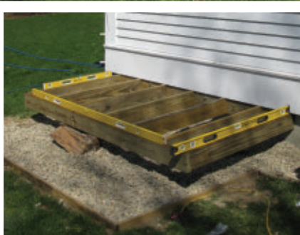
A gravel-covered base lined the foundation.
