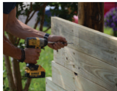
Attach the slats using quality exterior-grade fasteners, such as these #10 x 3" Spax HCRx coated screws.
