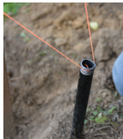
Tighten the string by wrapping it around the pipe threads and cinch it with a trucker's hitch. Brightly colored string offers high visibility.
