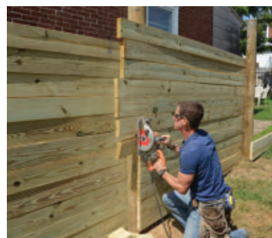
Snap a line and cut all the ends of the slats at once.
