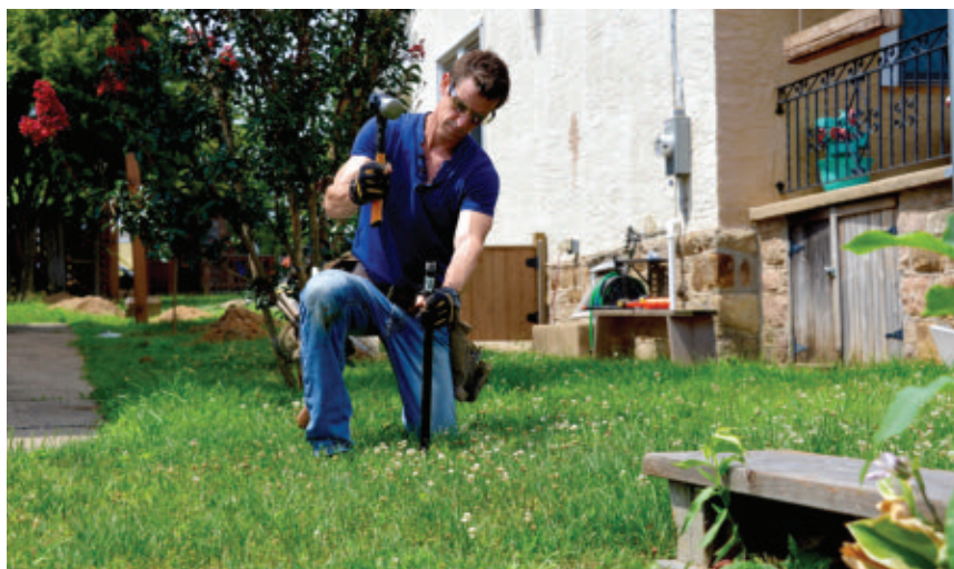
I map the layout by pulling string between lengths of gas pipe staked into the ground.
