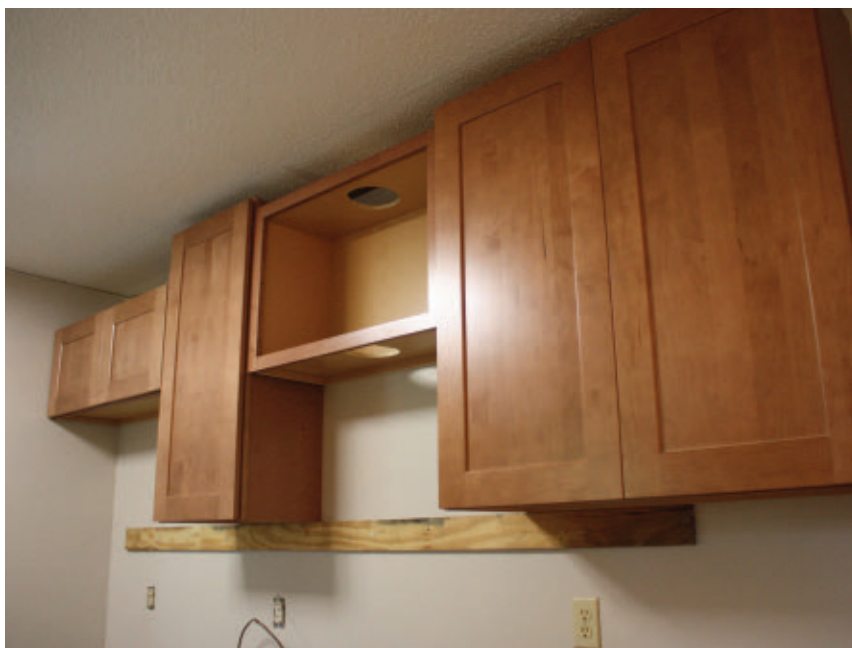
A temporary ledger board screwed to the wall along the layout line can assist in holding the cabinets while you install them.
