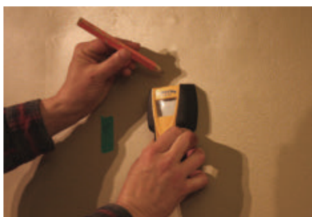
Locate and mark the wall studs.
