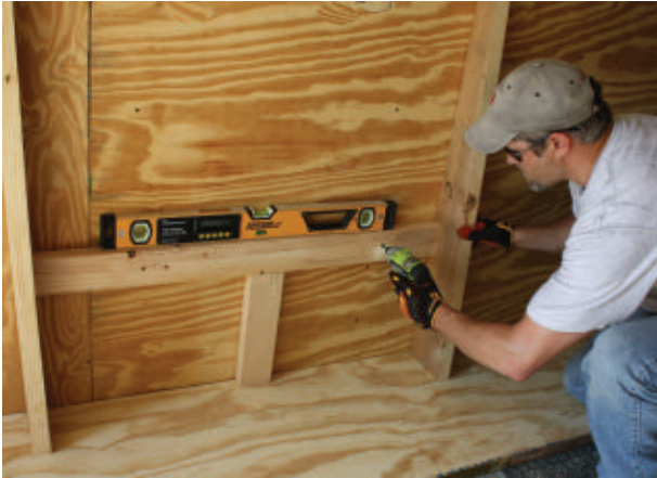
The horizontal cross-braces are mounted into the wall studs.
