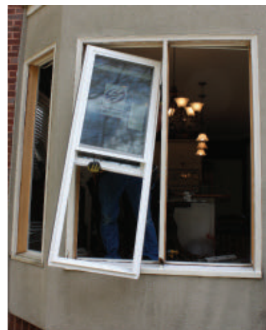
Because the installers were replacing the outer stop molding with aluminum casing, they opted to leave the interior stop molding in place and install the windows from the outside.
