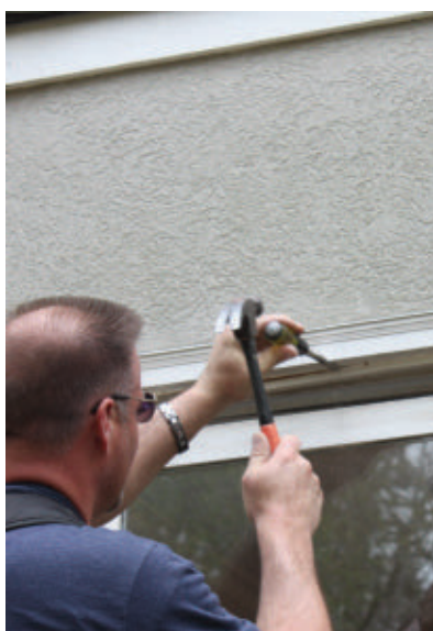
Stop molding surrounds the top and sides of the windows.
