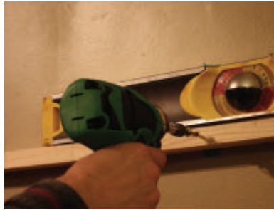
Level the cleat and screw into solid wall framing.
