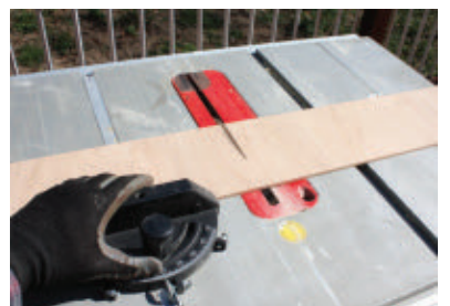
Trim the plywood to fit inside the groove.
