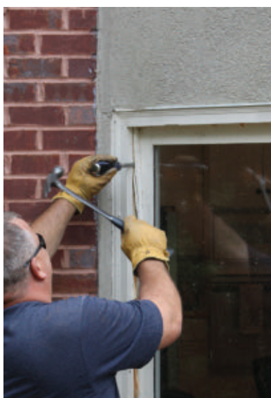
To remove the windows, remove the stop molding along the edges.
