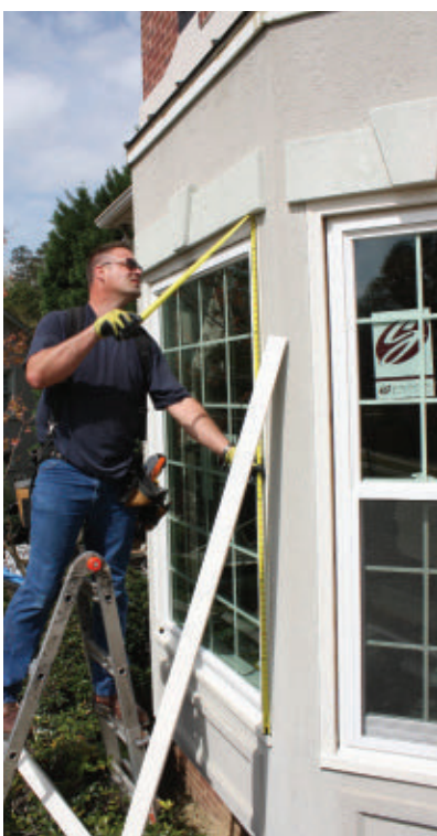
The windows are carefully measured to determine the length of the aluminum wrap.
