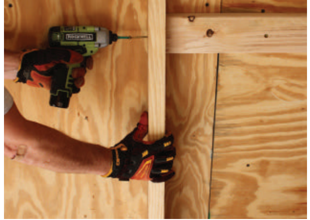
I mounted the angled supports with 3" screws driven into the end grain of the cross-braces.
