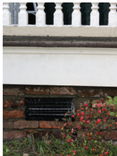
My house was built in the late 1800s, and in order to retain its historic character, I purposely did not fill-in and smooth out the grout lines of my brick with a striking tool.
