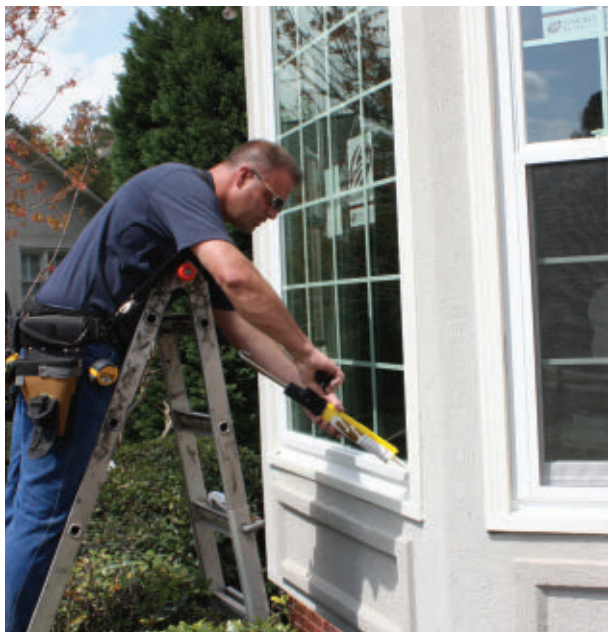
All seams of the window and aluminum casing are sealed with a high-quality exterior sealant.
