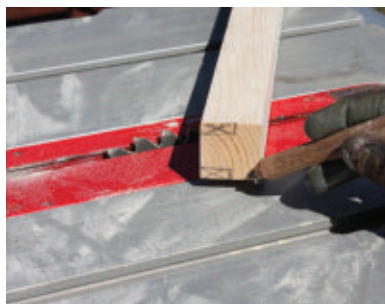
Measure and mark rabbets to seat the 1/4" plywood.
