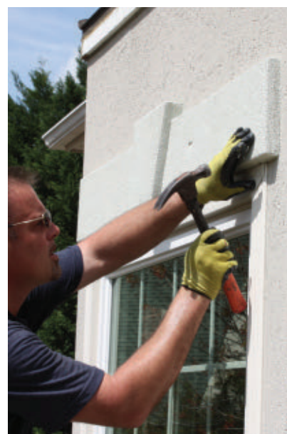
After the sides are wrapped, the final piece goes on top to divert water away from the building envelope.
