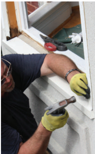
The sill wrap is the first piece to be installed so the window can be placed over it.
