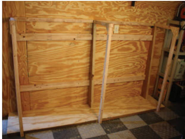
Before installing the top shelf I added 2x2 cross-braces flush with the tops of the angled supports.
