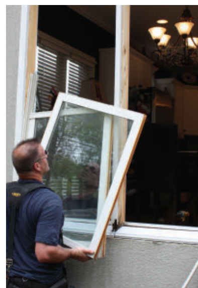
Once the stops are removed the windows can be carefully pulled out of position.
