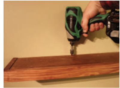
Fasten the shelf to the cleat with wood screws.
