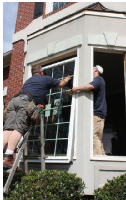
Large units require some assistance when installing. A worker on the inside lifts the window with a suction cup.
