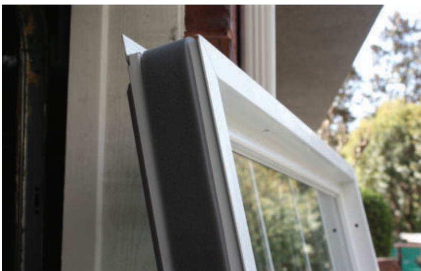
The Simonton windows arrive with weather stripping around the perimeter of the units. This helps the window to fit snugly, and adjustments to plumb, level and square can be made with wood shims.
