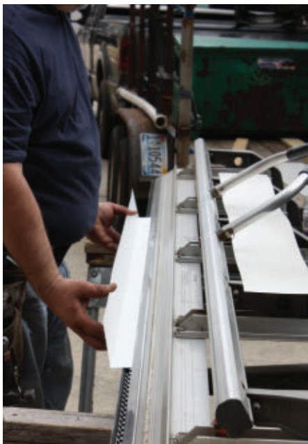
The aluminum trim wrap is fabricated on site to match the size and shape of the wooden window trim.
