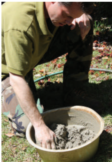
We mixed up small amounts of Sakrete masonry mortar in an old wash pan.
