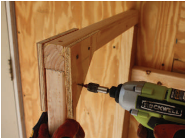
I installed the gussets on the L-brackets using a combination of deck screws and Gorilla Glue.
