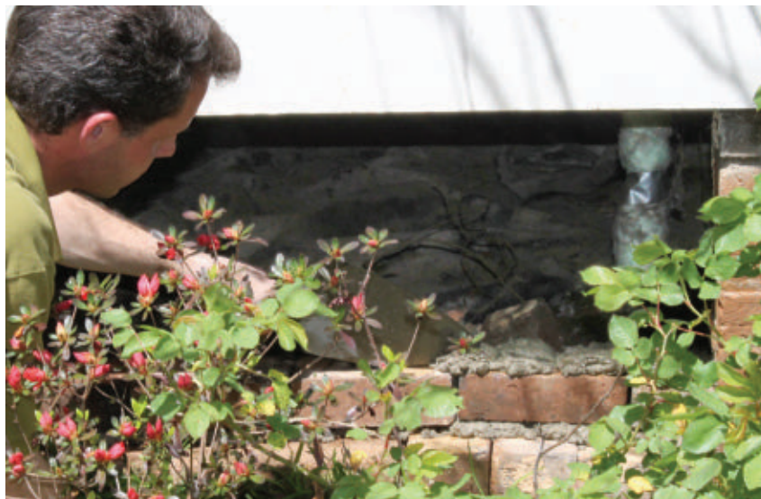
As I installed the rows of bricks, I placed the foundation vent in the middle of the section of brick and simply cemented it into place. The most difficult part of the masonry job was installing the top couple of rows above the vent because of the tight space.
