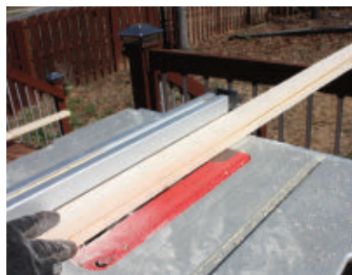
Make intersecting partial rips to cut the rabbets.
