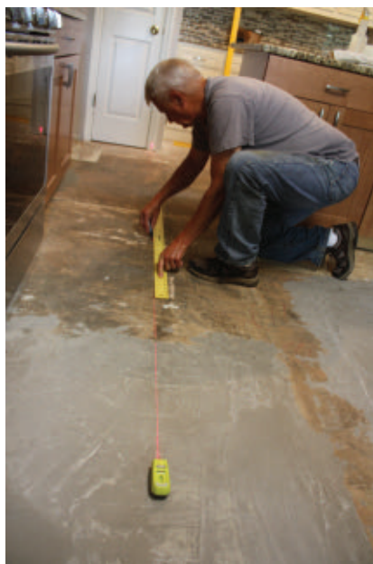
Begin your layout by marking crosshair layout lines that divide the room into quadrants.
