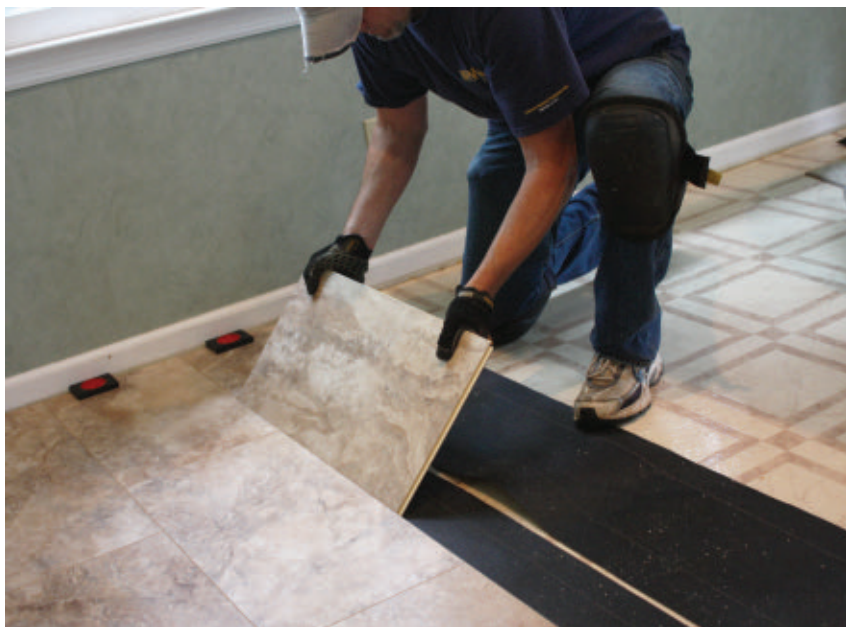
The luxury vinyl tile shown in this project clicked together with tongue-and-groove joints to form a waterproof floating floor. Here, we've moved from the kitchen into an adjoining breakfast room.
