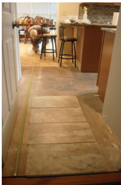
Take measurements from front to back and left to right to determine tile size along the edges of the room. Lay out a dry row of tiles for the best visual aid.
