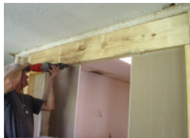
if you plan to widen a doorway or open a room's floor plan, you'll need to construct an adequately sized 2x header for any load-bearing wall.
