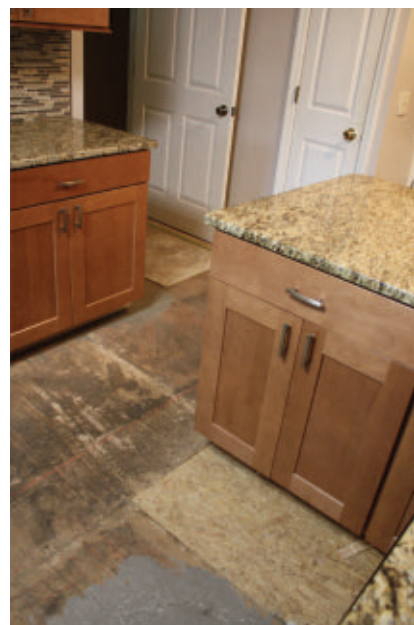
Rooms such as kitchens that are “chopped up” with lots of obstacles make tile-pattern layout a challenge.
