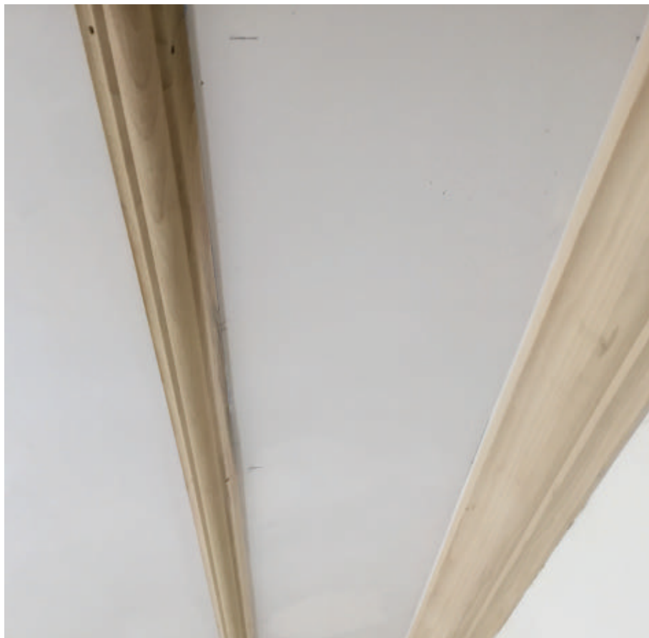
Astragal is installed 8" to 10" from crown.
