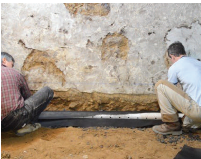
This is a good cross-section of a pipe going in. Because the entire floor was dug out here (for adding a bathroom), you can see the stone, pipe and fabric.
