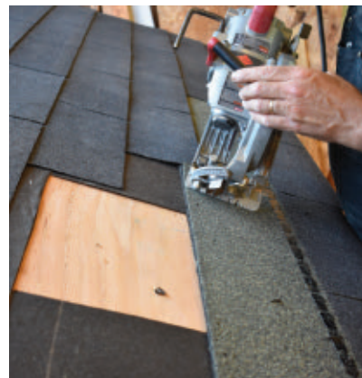
To install the brackets, remove roof shingles and cut through the roof deck above the exterior wall of the building.
