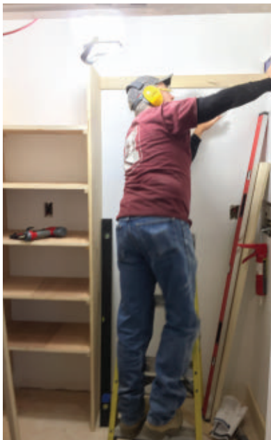
The top shelf is supported by a longer, wider cleat that is fastened to the wall studs.
