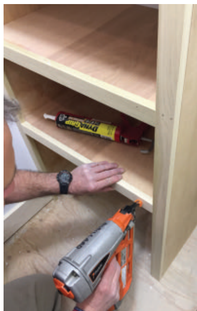
Fasten the face-frames and nosing with combination of glue and finish nails.
