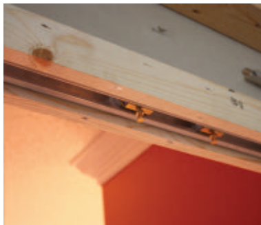
Slot the wheel hangers into the metal header track.
