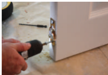
Screw the lock tabs to the door 2" from each edge.
