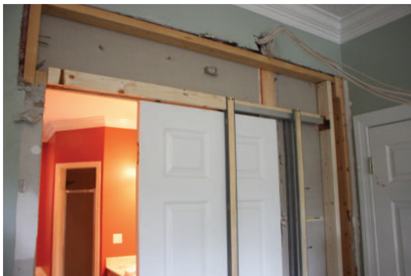
Metal lock tabs are mounted to the top of the door will connect to the hangers.
