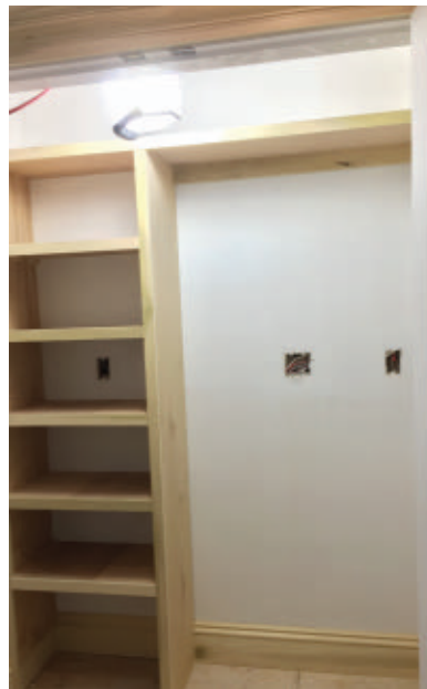
A baseboard installed at the bottom helps to stabilize the middle panel on the backside.
