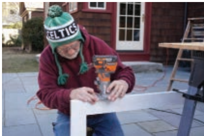
A trim router makes short work of the mortise.
