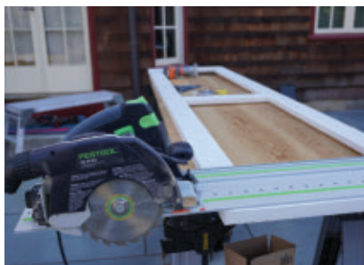
Use a circular saw with a rip guide to ensure straight cuts on the door frame.
