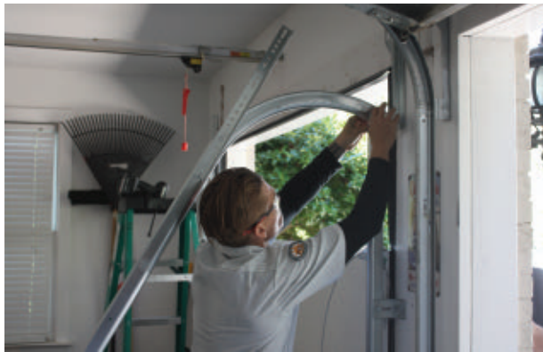
The ceiling tracks are curved to fold the door panels as they rise.
