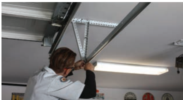
The ceiling tracks are suspended by slotted angle brackets mounted to the ceiling. The workers were able to reuse the existing angle supports left from the old garage door.
