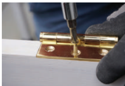
Avoid using a power drill on brass screws and instead tighten them by hand with a manual screwdriver.
