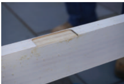
The trim router and a wood chisel leave shallow but accurate cuts for the recessed hinges.
