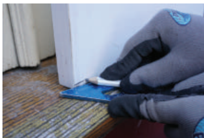
Mark the reveals of the door and make any final adjustments so the doors fit.
